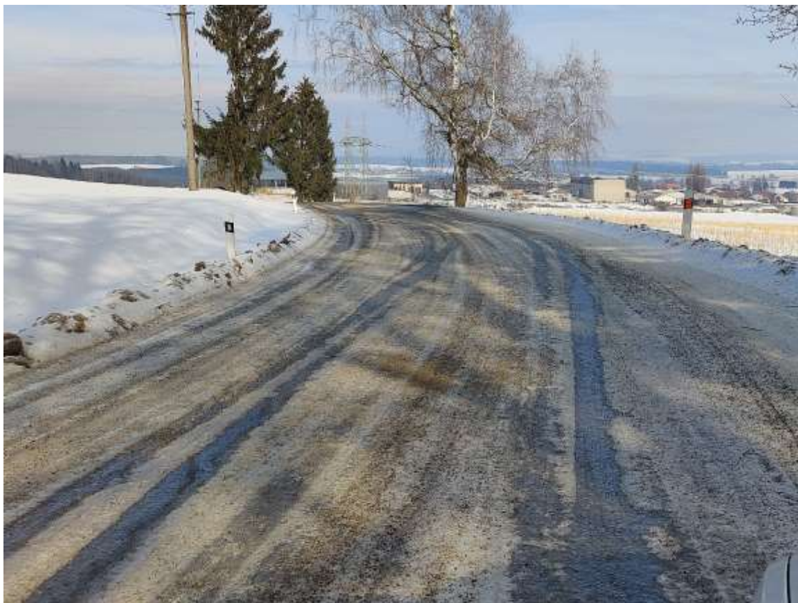
Figure 1 – Example of a section with abrasive treatment
