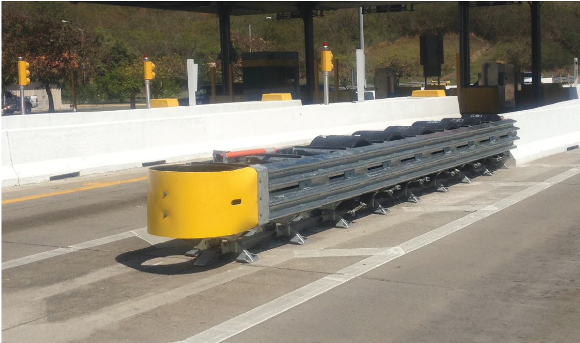
Figure 3.1 : The QuadGuard® Elite ; a redirective, non-gating crash cushion [12]
