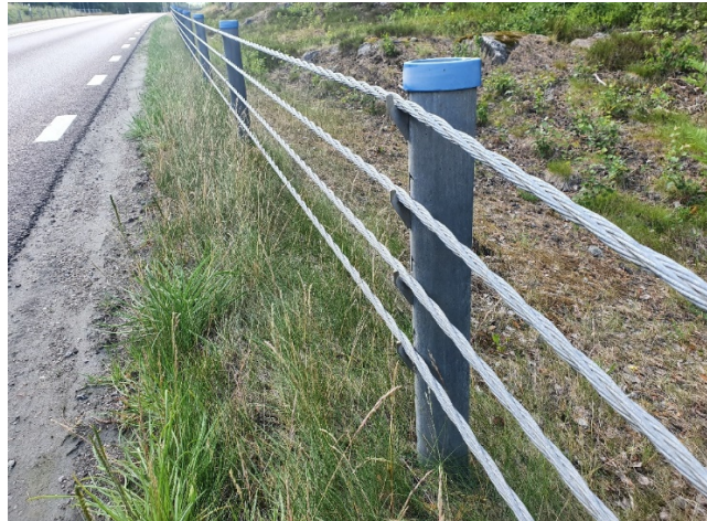
Figure 3.40 : Flexible cable barrier - "rope barrier"; Sweden
