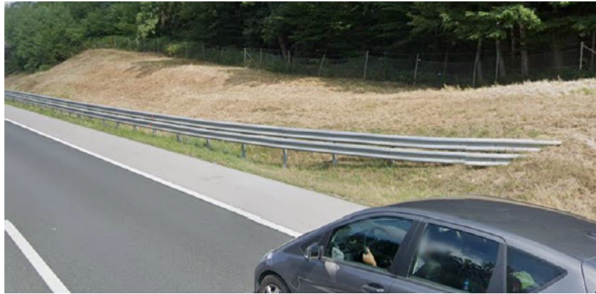
Figure 3.15 : SSB guardrail finished into embankment - example
