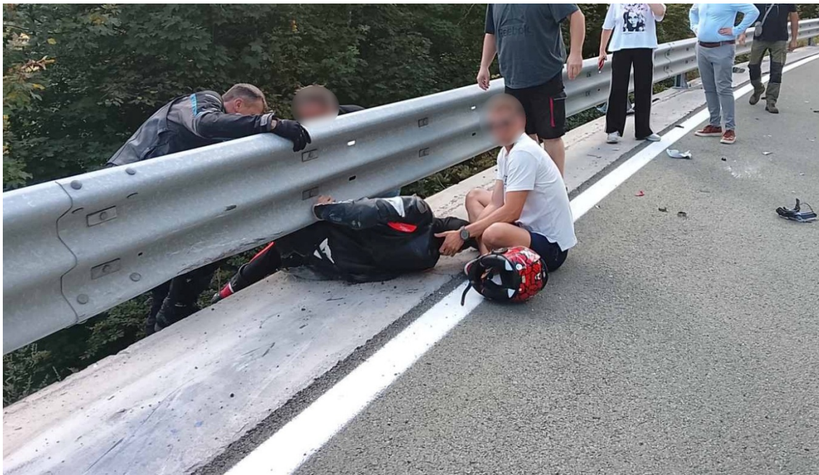
Figure 3.16 : Motorcyclist sliding under the barrier and impacting the post of a SSB
