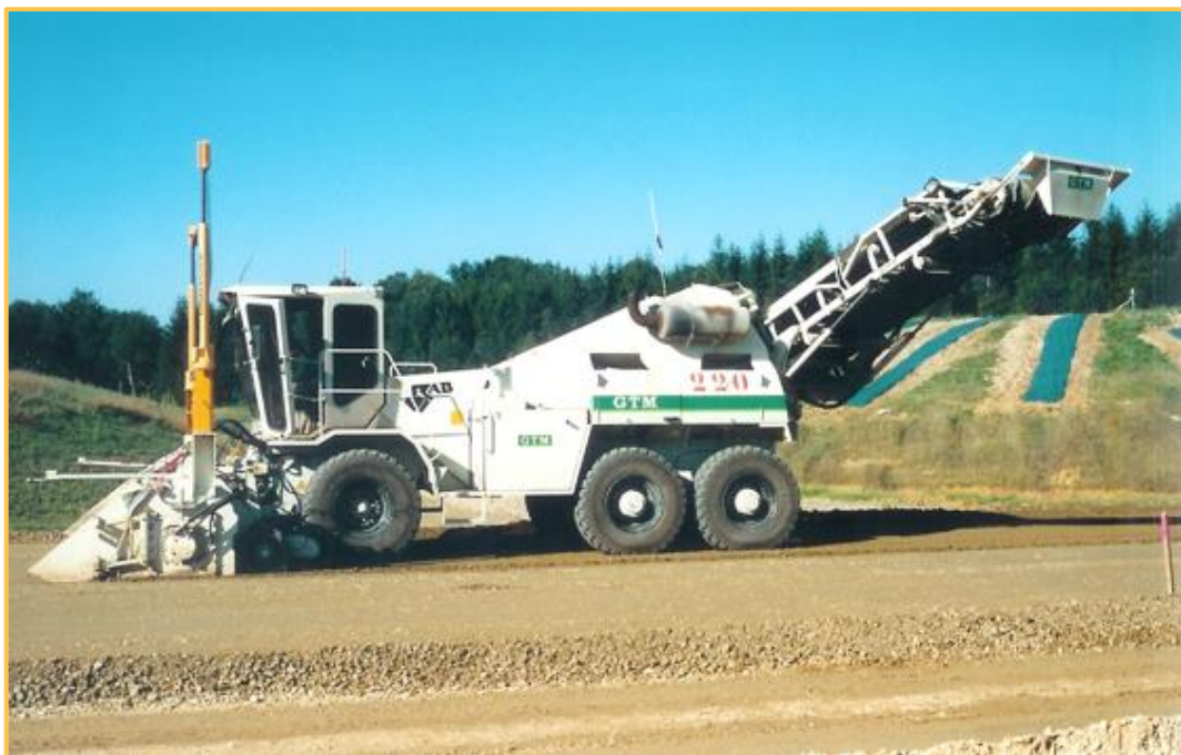
(2) Rotograde RABAUD/GTM (Photo GTM Terrassement) Picture 48: Construction site Capping layer / Grading Rotograde
