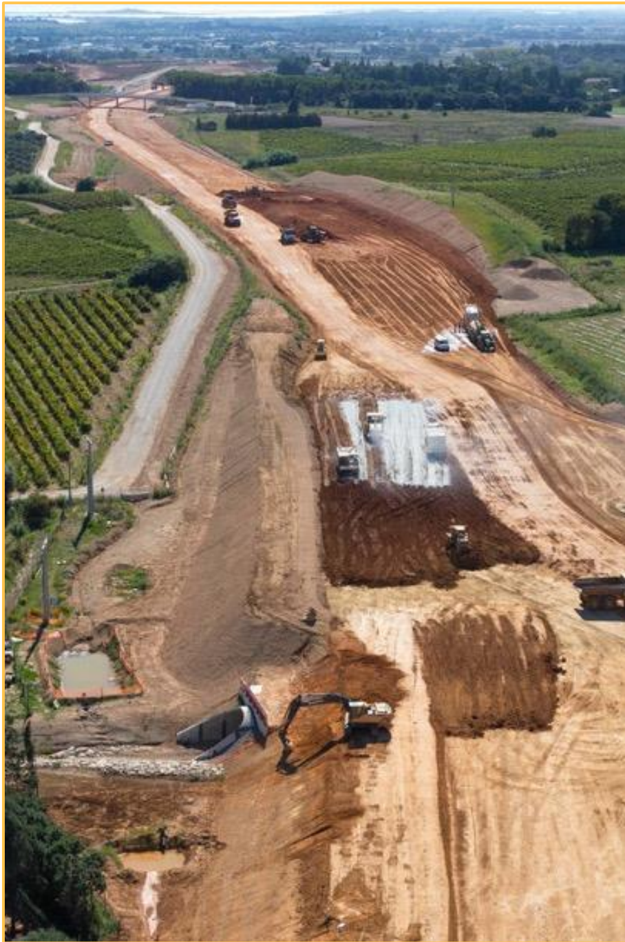
Motorway A9 Montpellier France (Photo VINCI Construction Terrassements) Picture 39: Treatment on the fill
