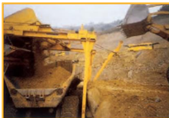
Ejection of coarse elements by tilting the grid actuated by the loader bucket during its reverse gear.
