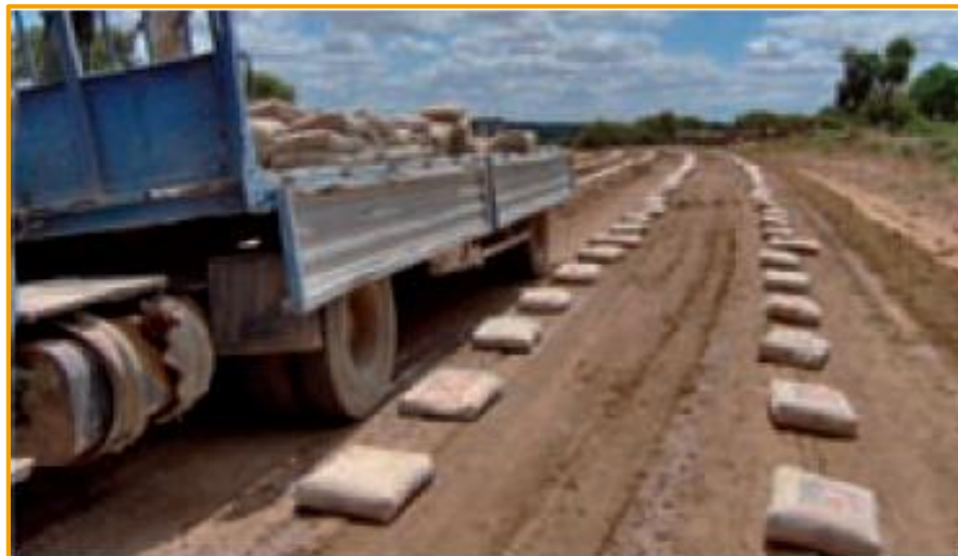
Picture 11: Bag spreading (Photo CIMBETON)
