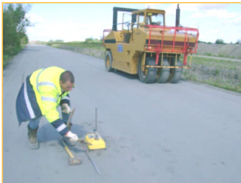
Construction site capping layer in treated fly ash LE HAVRE Recommended compaction with tyred roller / Checking the density with a gammadensimeter Picture 46: Job site Capping layer / Final compaction heavy pneumatic tyred rollre (Photo GTM Terrassements)
