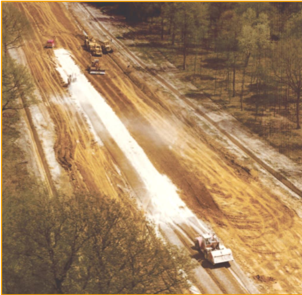
Picture 1: Lime treatment of fill [A36 Beaune-Dôle (1980)]
