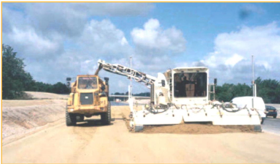
(1) (1) Grading of the capping layer with Rotograde 2000 (Photo GTM Terrassement)
