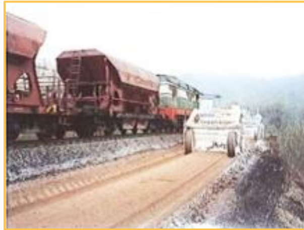
Lime treatment of the TSE of a railway track (reconstruction of a second track) Picture 25: Embankment in confined area
