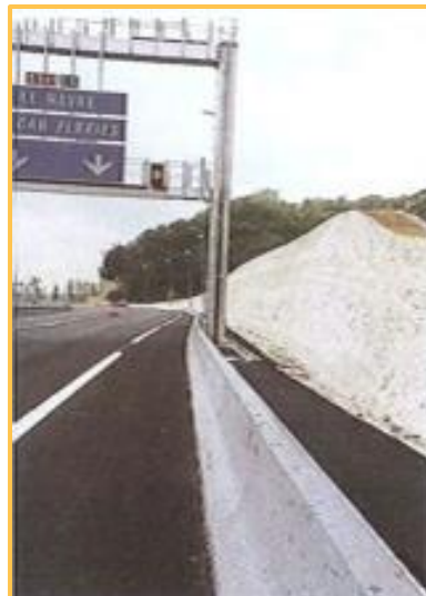
Sides of cut in silt supported with hydraulic binder stabilized chalk (Photo GTS) Picture 26: Slope stiffening
