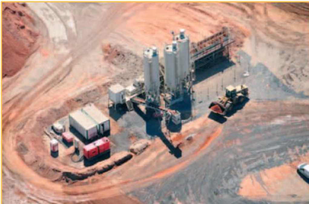
RN 33 France Treatment plant with hydraulic binders / Sand and fly ash mixtures (Photo GTM Terrassement)
