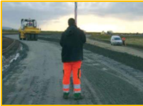
Surface closure by pneumatic tyred roller and topographic reception
