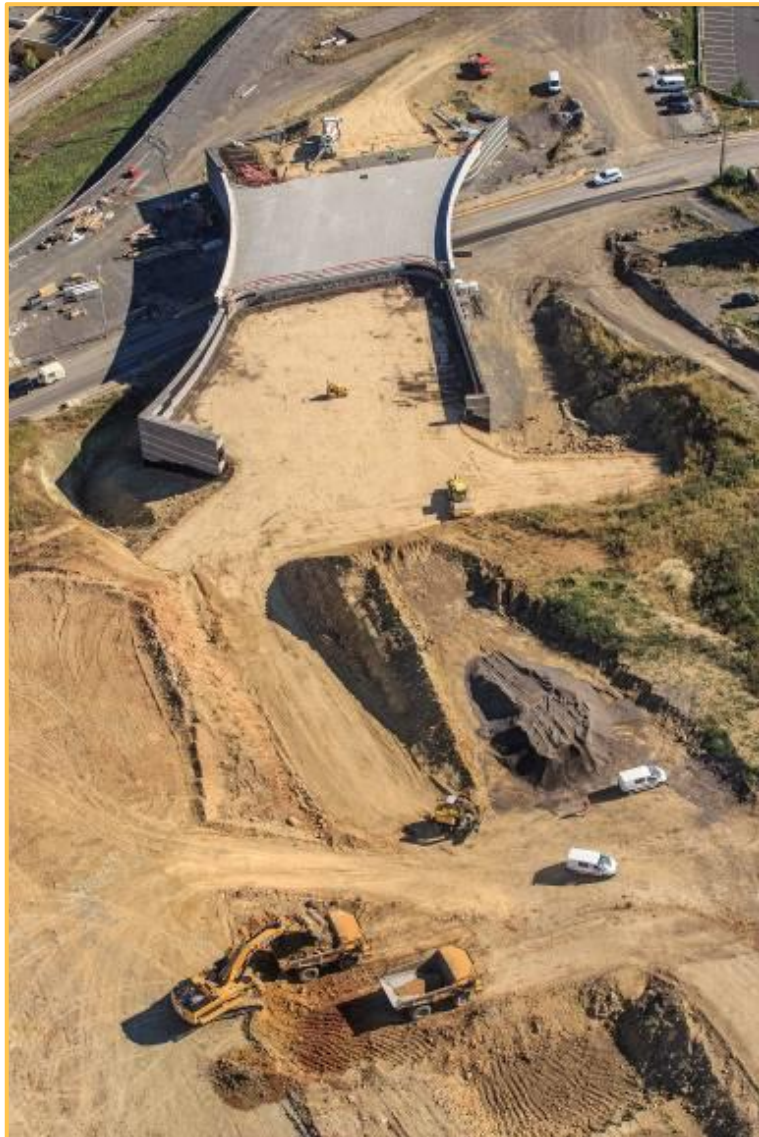
Picture 5: Embankments adjacent to the works (RN 88 LE PUY – Crédit RAZEL)
