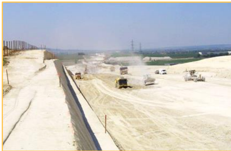
Picture 7: Masks Lot 22 TGV East (chalk treated with 7% HRB)
