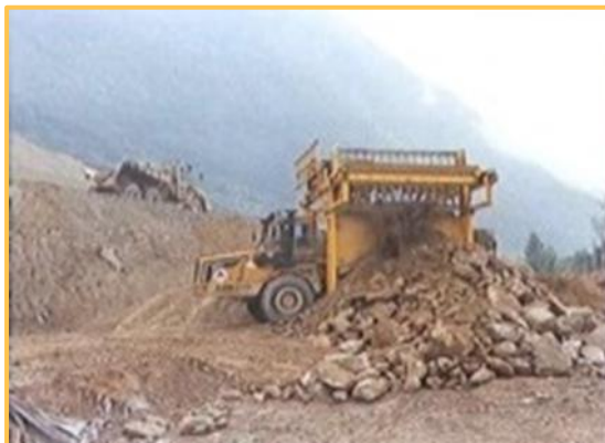
Screen and oversize blocks dumped aside.
