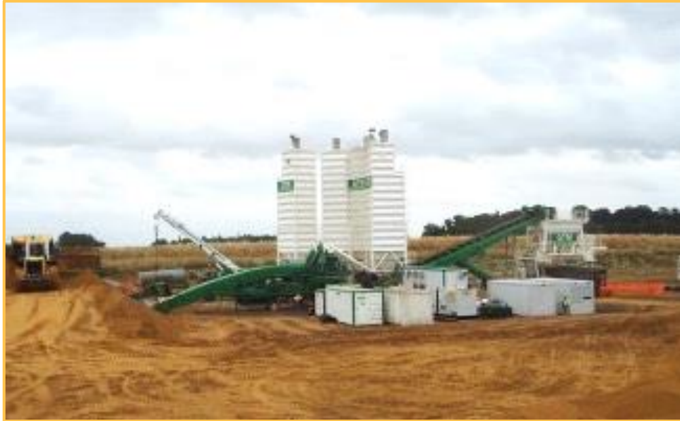
Picture 17: Mixing plant / Treatment of silts with binders for capping layer (Photo GTM Terrassement)
