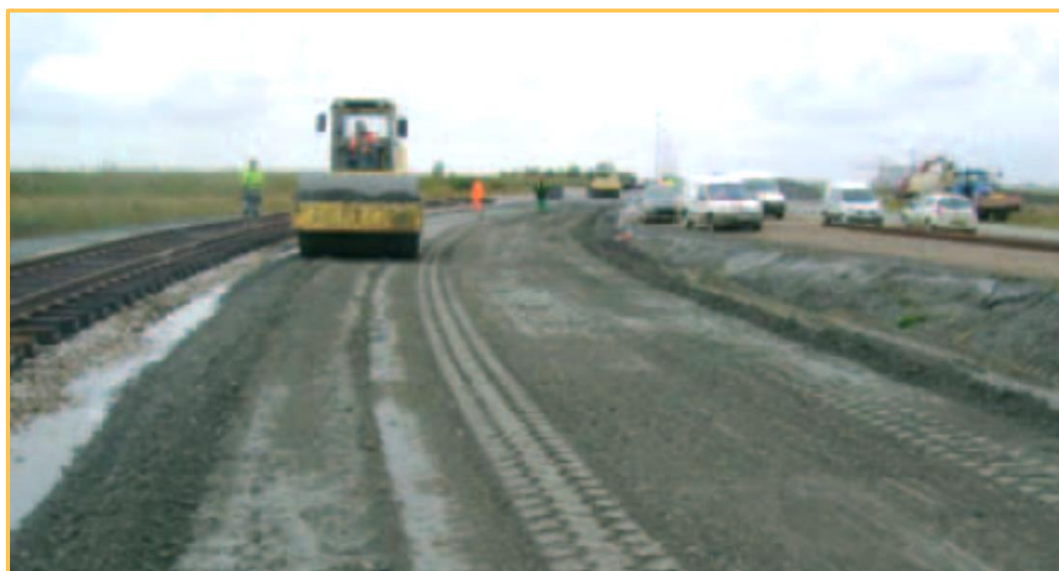
Picture 2: Capping layer made of treated fly ash
