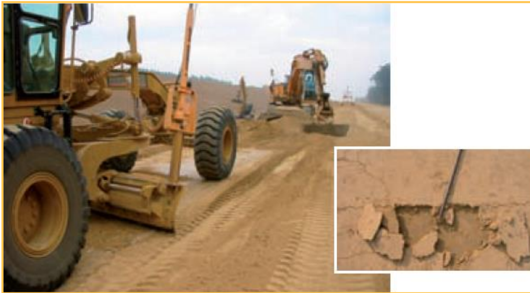
(1) Grading capping layer with a grader (Photo CIMBETON)
