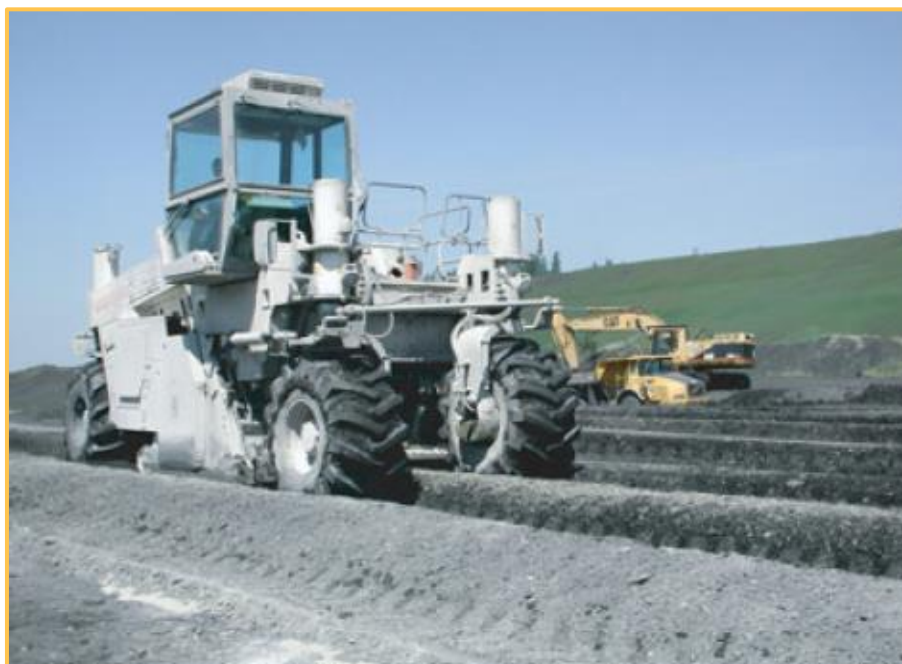
Dourges jobsite France (Photo Razel) Picture 36: Binder Mixing Plants
