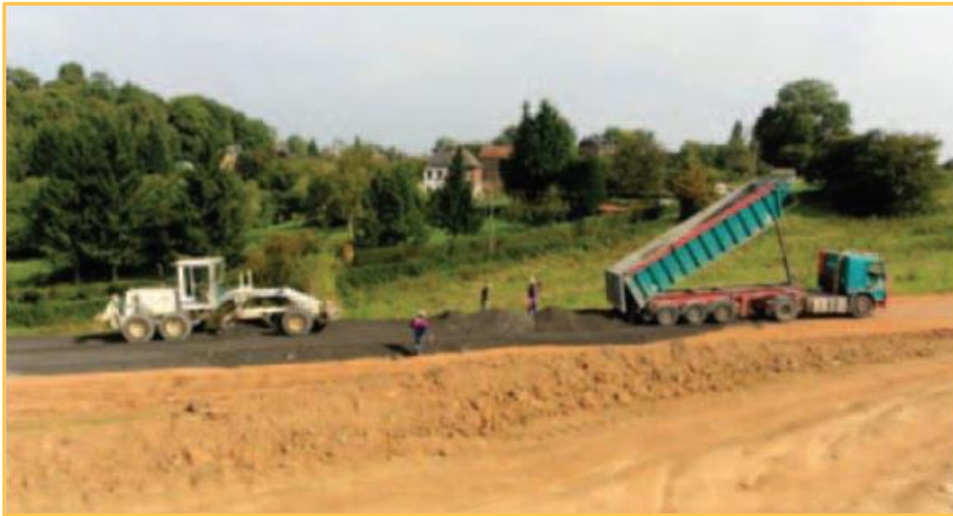
Picture 3: Creation of a gravel capping layer from recycled non-hazardous waste incineration slag
