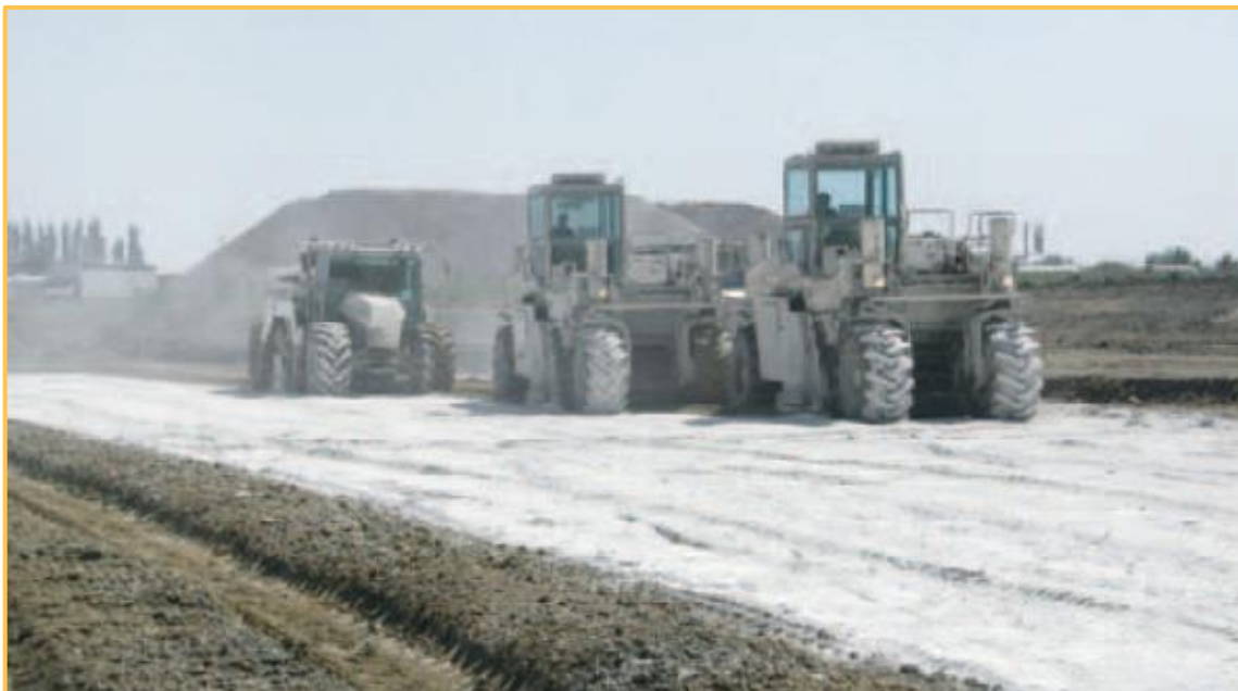
Picture 4: Treatment of coal shale with hydraulic road binder (Dourges logistics platform Delta 3 (2002))
