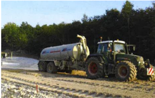
Carp tail sprinkler (photo NGE)
