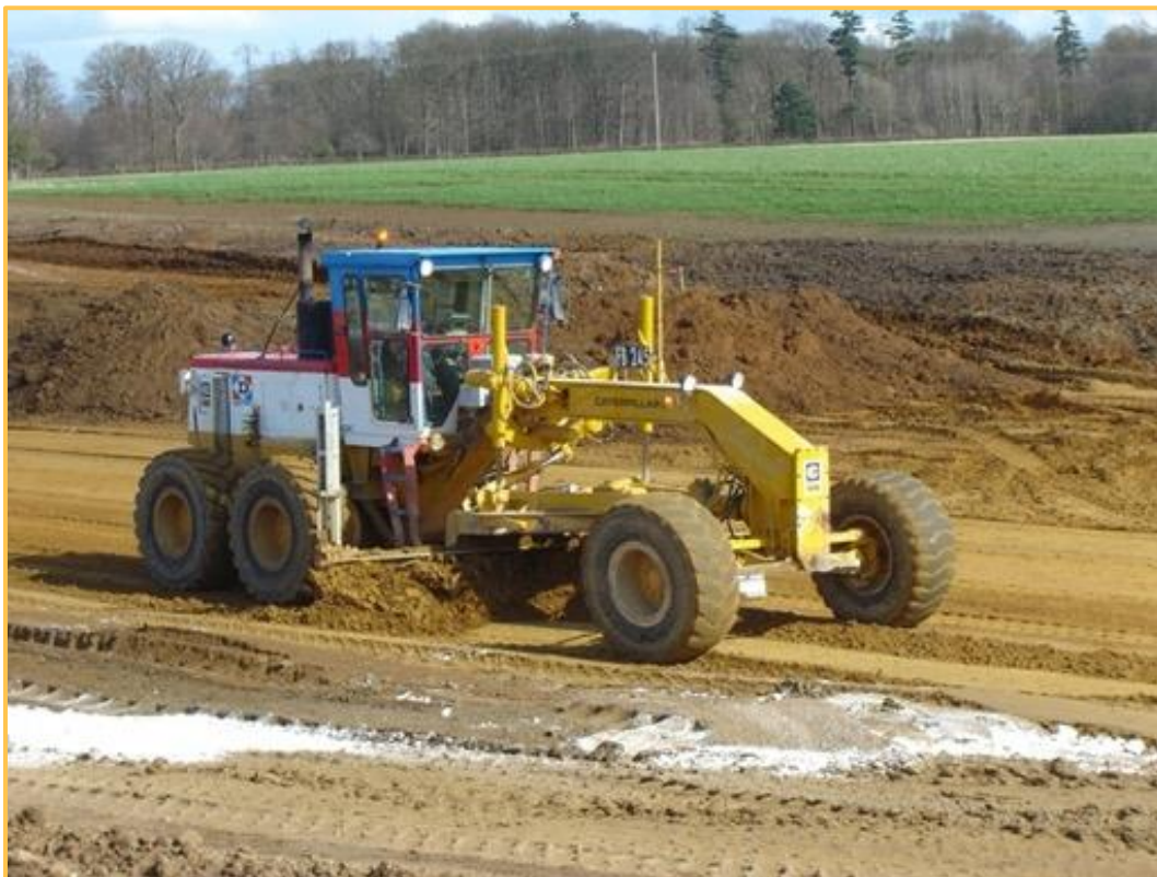
(2) Grading with a grader (Photo DTP Terrassement) Picture 47: Job site Capping layer / Grading workshop
