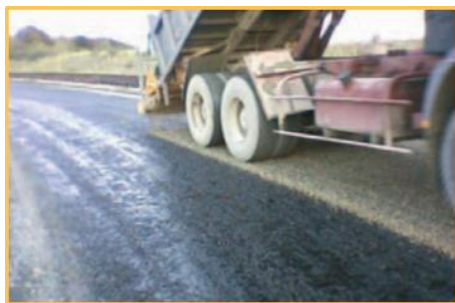
Picture 49: Job site Capping layer / Surface protection
