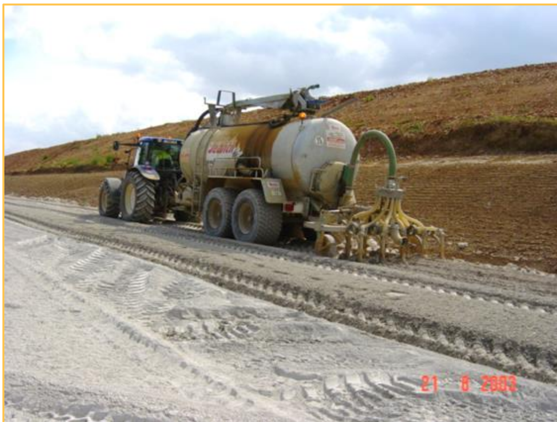
Motorway A89: Capping layer in treated silts (photo RAZEL) Humidification with burying sprinkler Picture 43: Capping layer Job site with humidification
