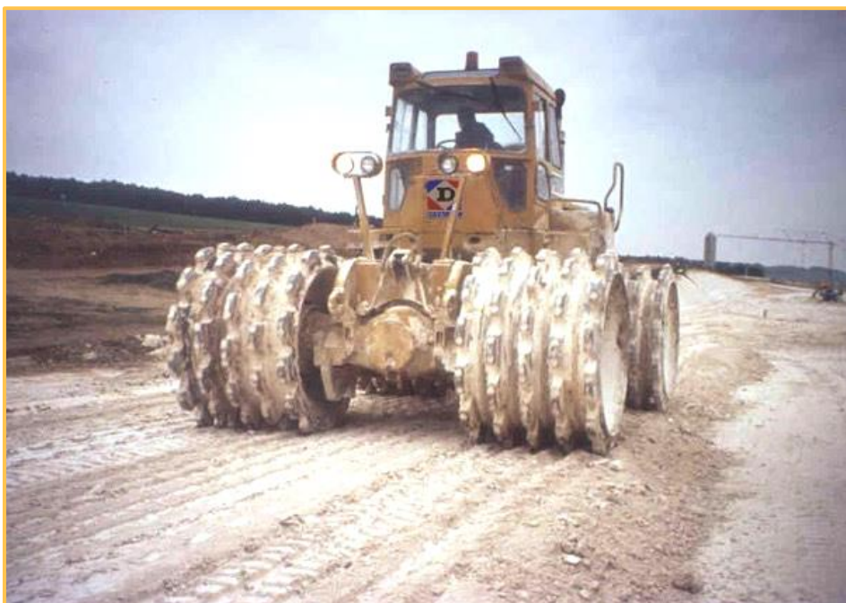
Picture 23: Tamping (Photos DTP Terrassements)
