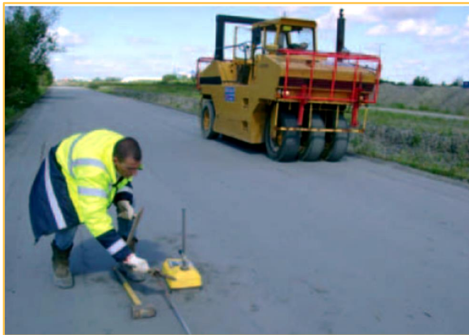
Picture 22: Pneumatic-Tyred Roller (Photo GTM Terrassements)
