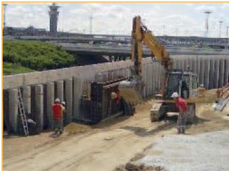
Picture 5 bis: Example of use of lime treated materials as embankment behind a structure (Copyright Guide Matériaux chaulés)
