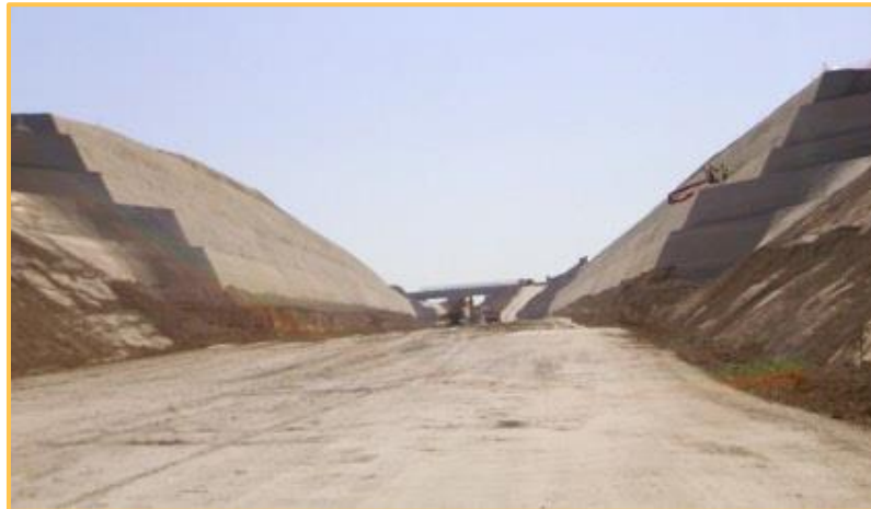
Picture 6: Masks Lot 22 TGV East (chalk treated with 7% HRB)
