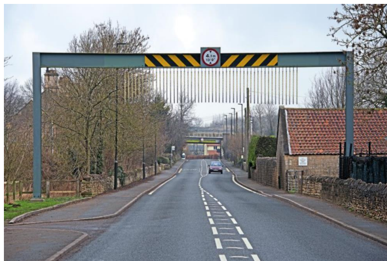
Figure 4.3: Hanging chains for preventing bridge strikes (Railway Magazine, 2021).
