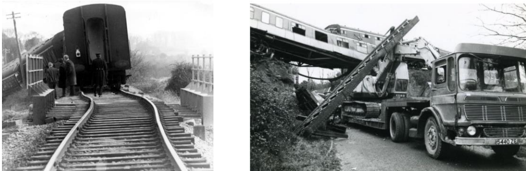
Figure 4.7: Train derailment at Longford 1974 (left) and Wexford 1975 (right) due to undetected bridge strikes (Byrne 2009).
