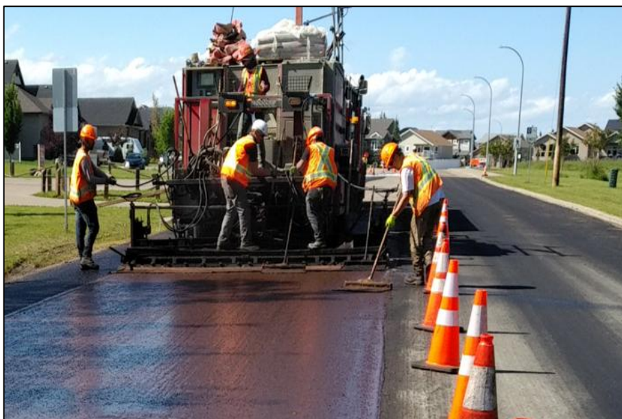
Figure 4. 7: Application of a Microsurfacing low-volume rural road (Reference: Red Deer )
