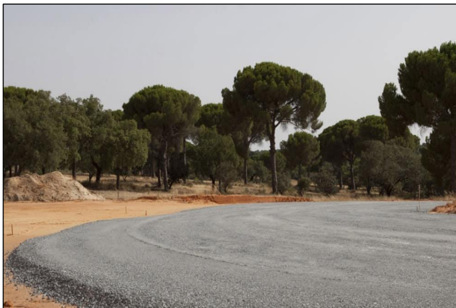
Figure 4. 5: Construction of a Bitumen stabilized low-volume rural road (Reference: Globalroadtechnology )
