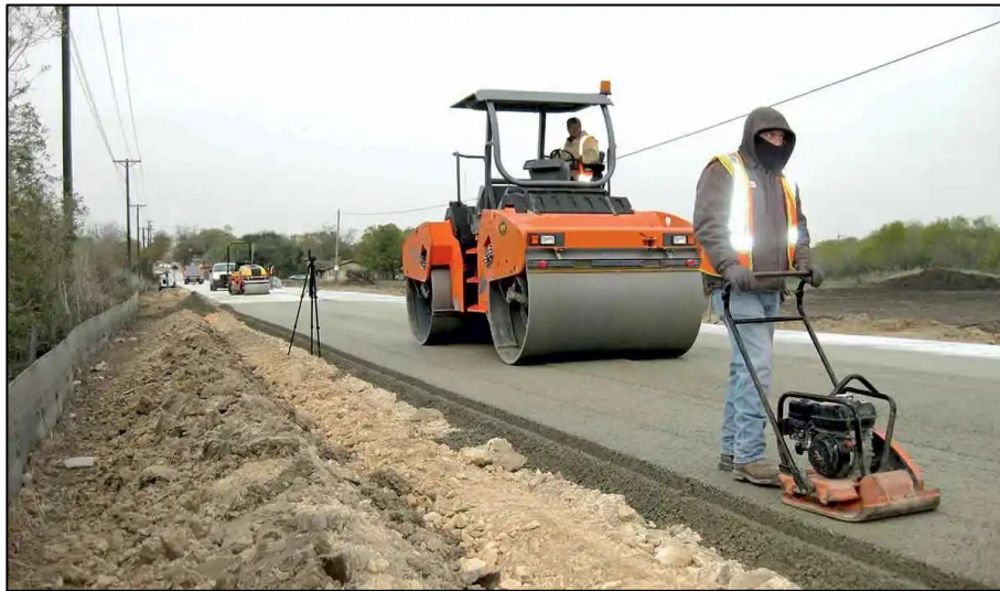
Figure 4. 14: Construction of a RCC low-volume rural road (Reference : Green Tech Programme )
