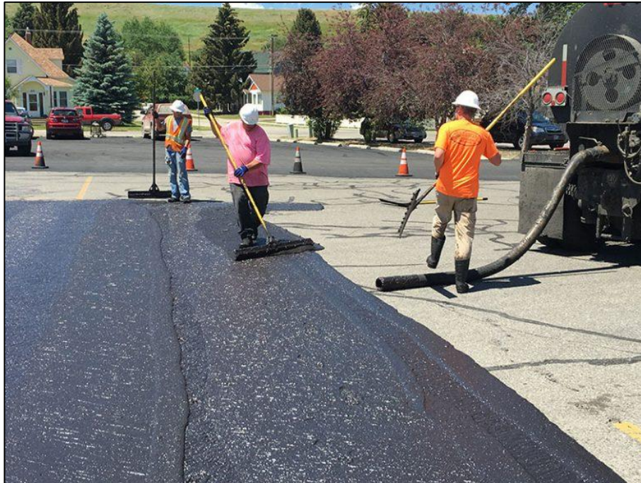
Figure 4. 8: Application of a Slurry seal low-volume rural road (Reference: Bitumen6070 )
