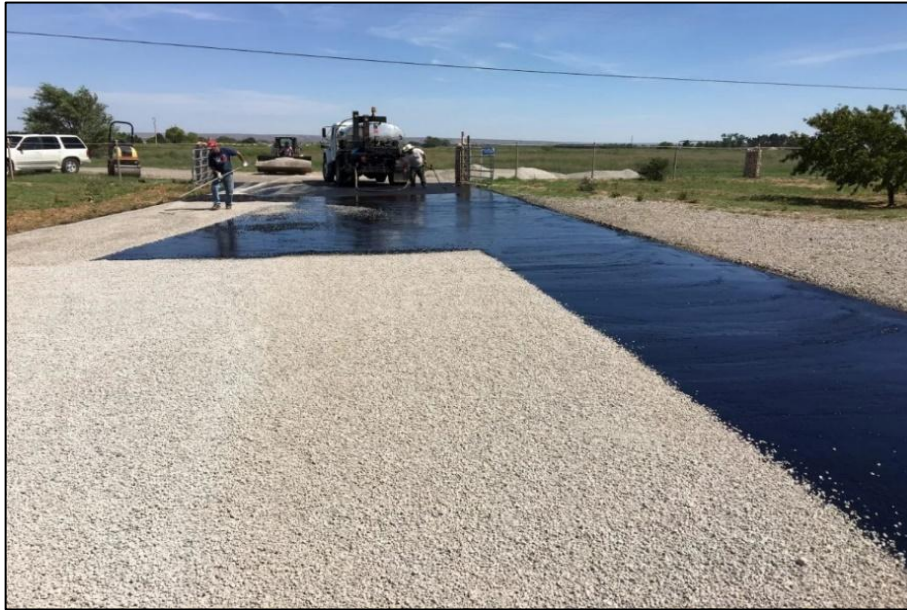
Figure 4. 6: Application of Chip Seal on a low-volume rural road (Reference: Driveway Experts )
