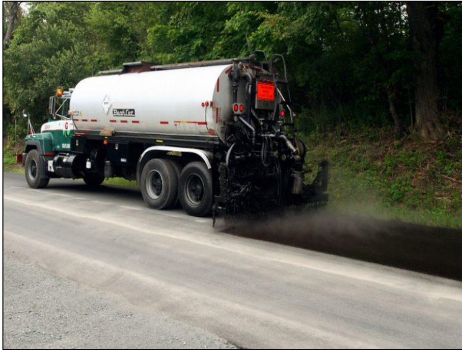
Figure 4. 9: Application of a Fog seal low-volume rural road (Reference : Rahabitumen )
