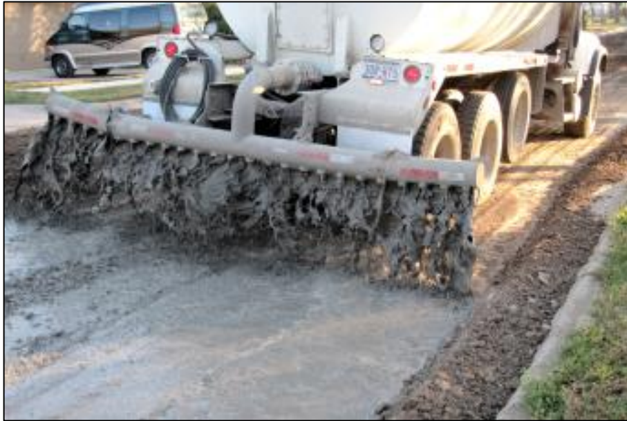
Figure 4. 3: Construction of a Cement stabilized low-volume rural road (Reference: Matinmarietta )
