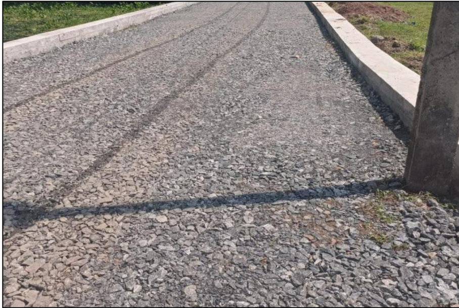
Figure 4. 2: Wet Mix Macadam Road (Reference: Rebuild Kerala Initiative )
