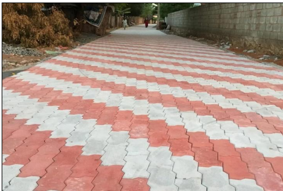
Figure 4. 12: Concrete paving block pavement (Reference : Jontypavertiles )
