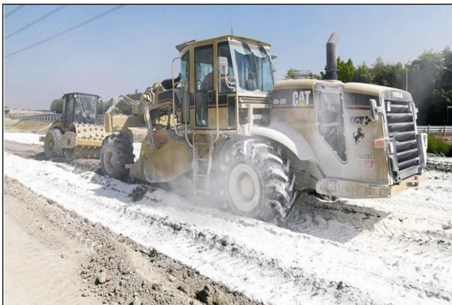
Figure 4. 4: Construction of a Lime stabilized low-volume rural road (Reference: Civilengineersforum )
