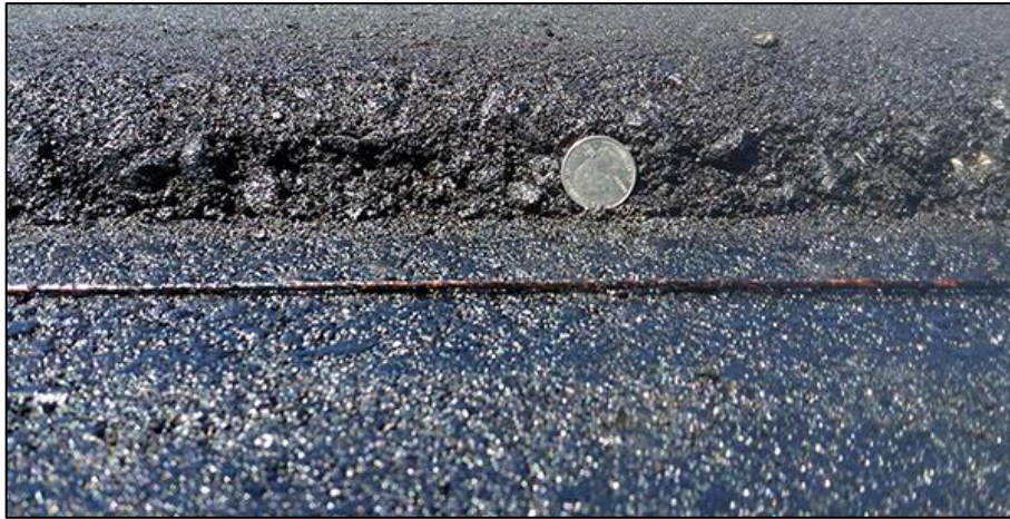
Figure 4. 13: Construction of a Thin bituminous surface (Reference : asphaltmagazine.com )
