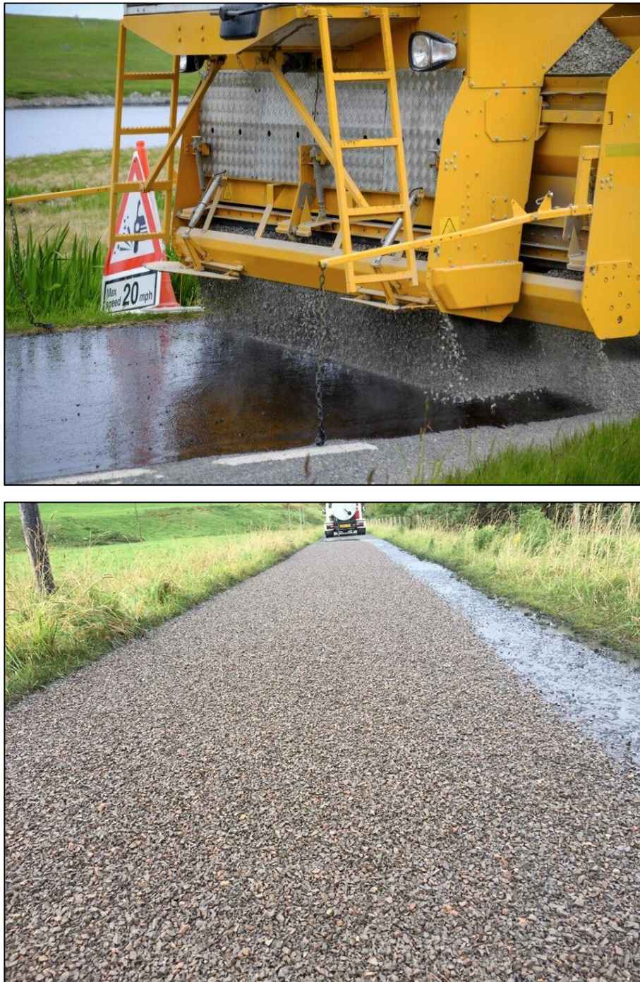
Figure 4. 10: Application of a Surface dressing low-volume rural road (Reference : Colas (top) and Northumberland Surfacing (bottom))
