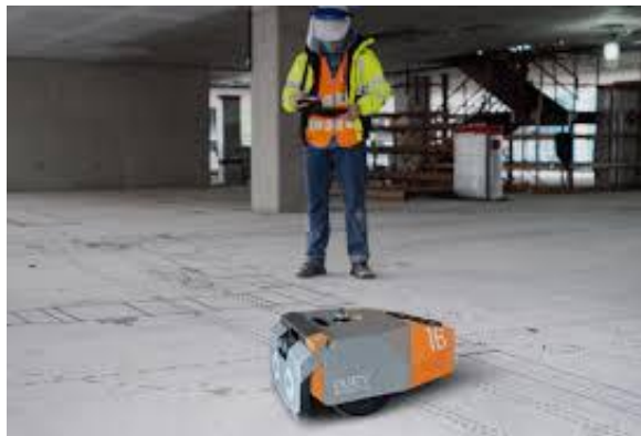
Figure B.20: AI-powered robotic systems automate the layout and marking of construction sites with high precision, reducing manual labour, minimising errors, and speeding up the process (Dusty robotics, 2024).
