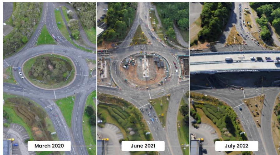
Figure B.15: A46 Binley project. Sensat's timeline feature used for remote progress monitoring during construction (Sensat, 2024).
