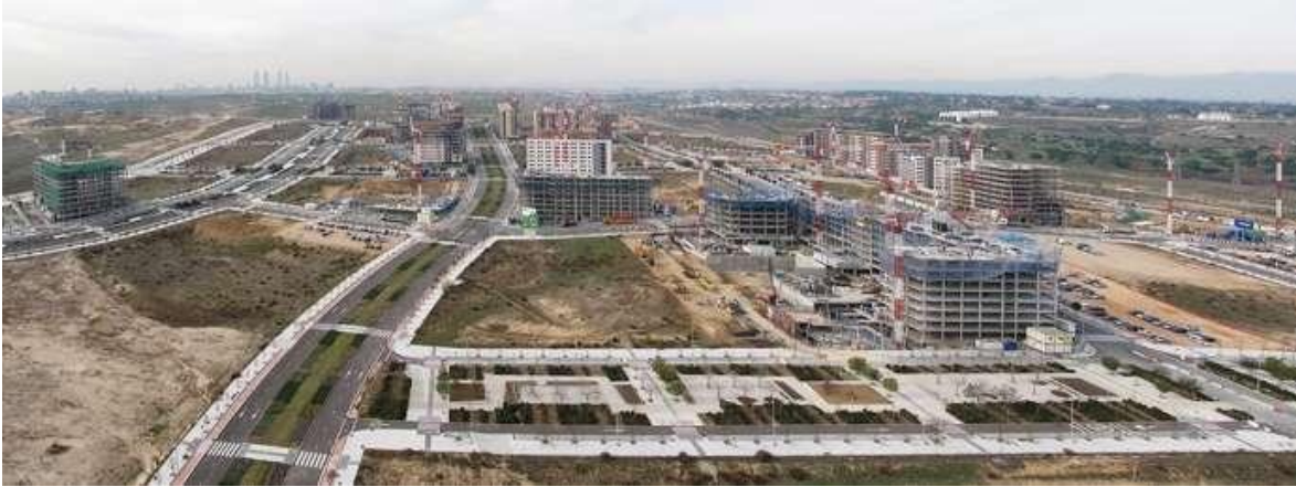
Figure 31. Change in land use: new urban infrastructure and buildings will modify runoff coefficients and the interaction of the road with its surroundings.
