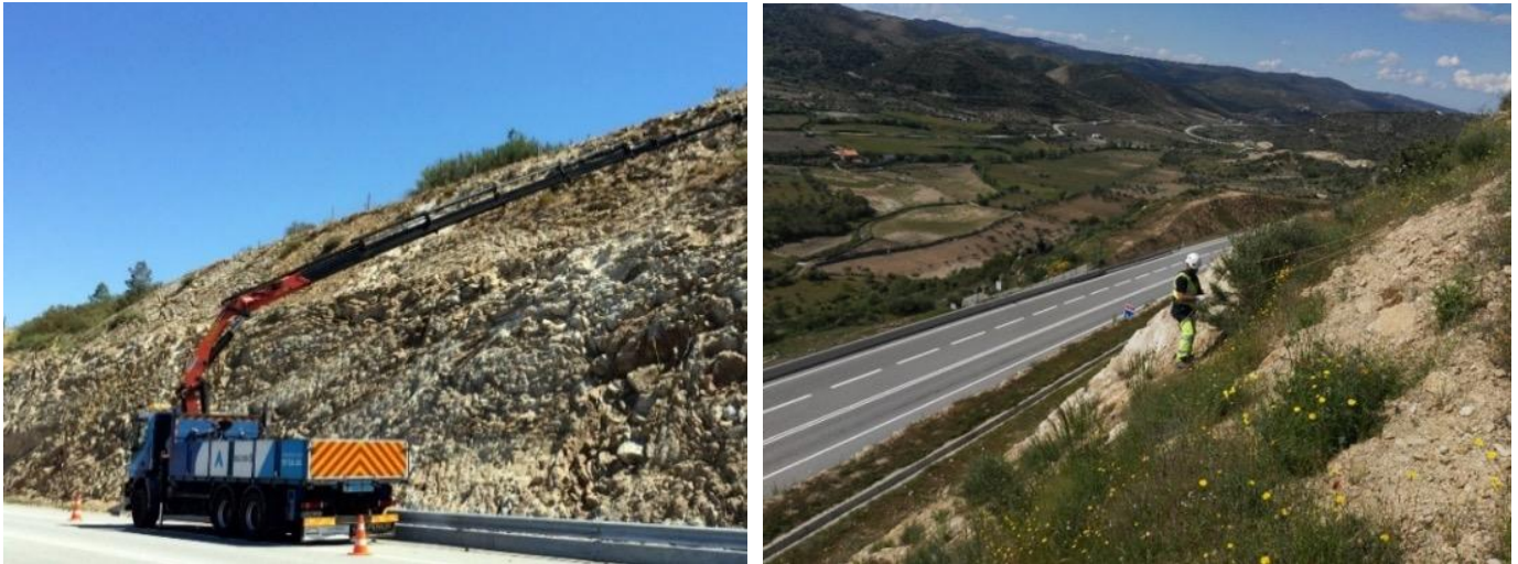
Figure 28. Checking condition of slopes
