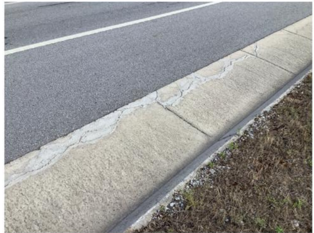
Sealing of cracks in drainage channel
