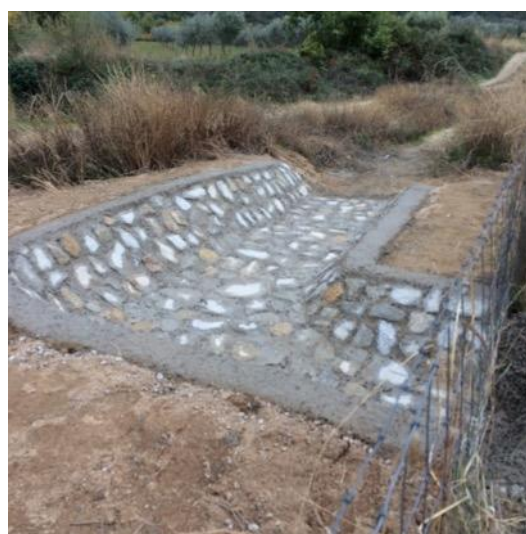
Reconstruction of drainage gully
