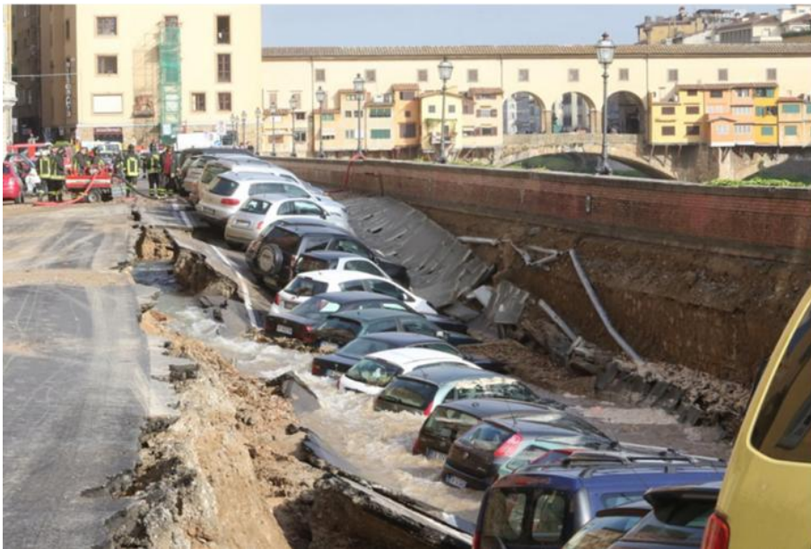
Figure 11. Lungarno riverfront road collapsed behind a retaining wall due to huge sewer leakage. The famous 'Ponte Vecchio' in the distance (Florence, Italy)
