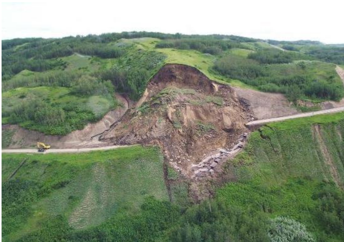
Figure 8. Huge landslide (Canada)
