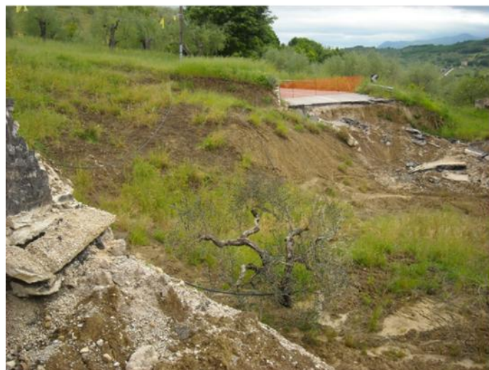
Figure 7. Embankment completely destroyed by a landslide (Southern Italy)
