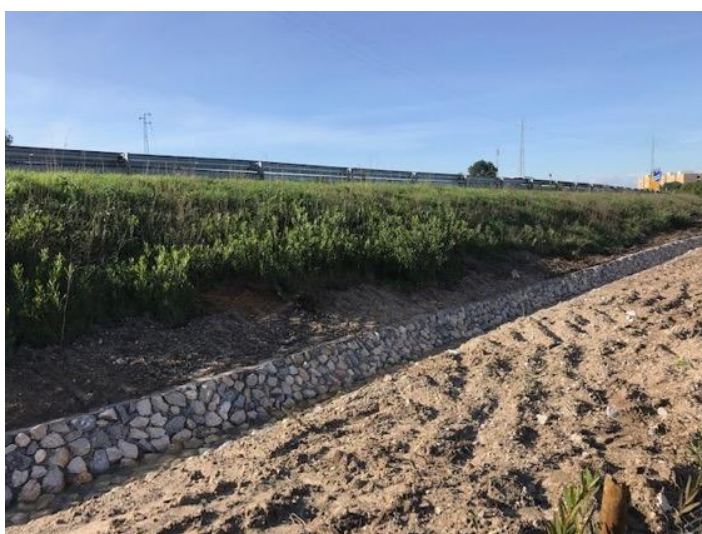
Repair of foot ditch of talude
