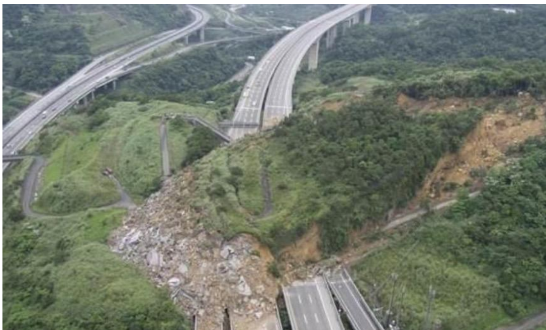
Figure 9. Highway cut by a landslide
