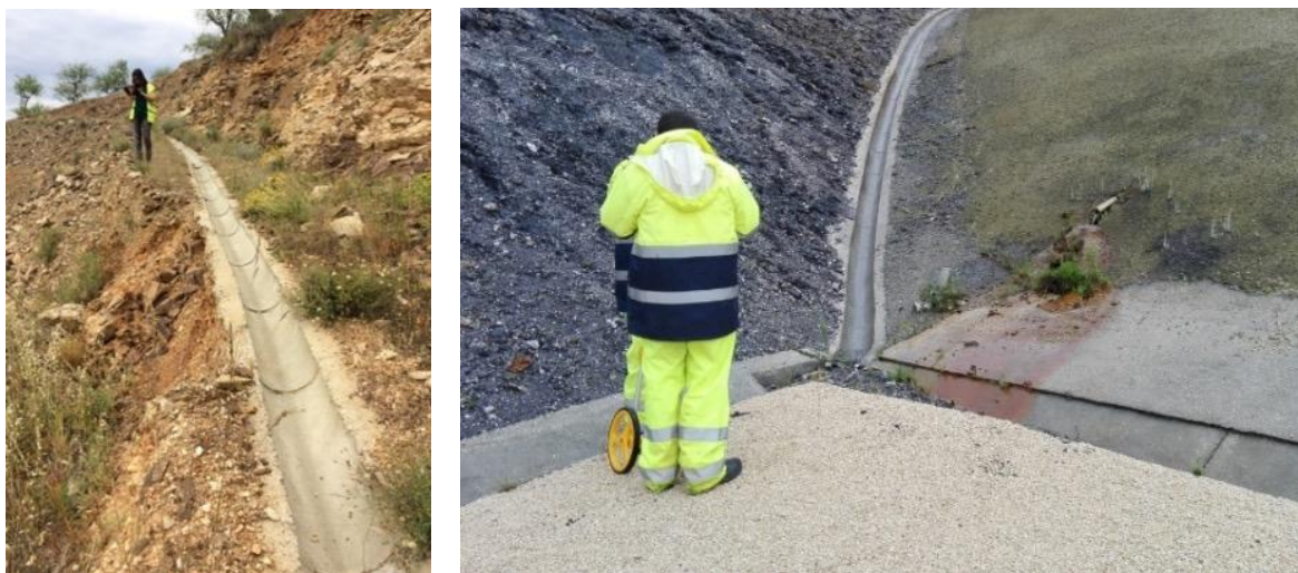
Figure 27. Checking condition of drainage lines
