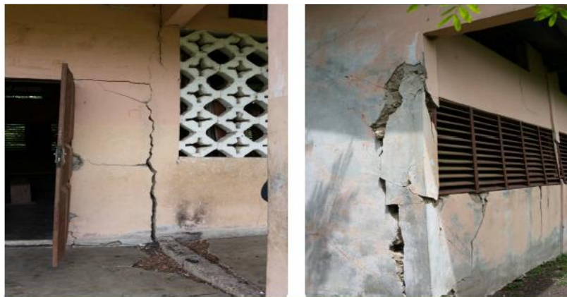
Figure 13. Effects on buildings of soil settlement/rising due to temperature variations (Houeyogbe, Benin)
