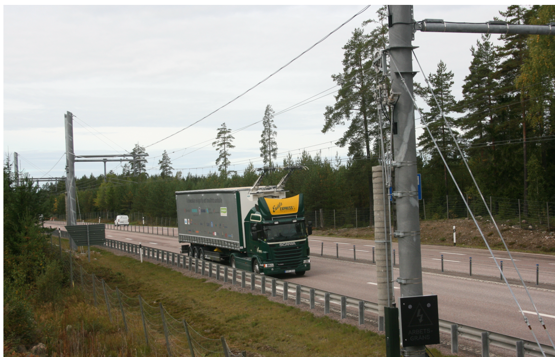
Figure 16. eHighway in Sweden
