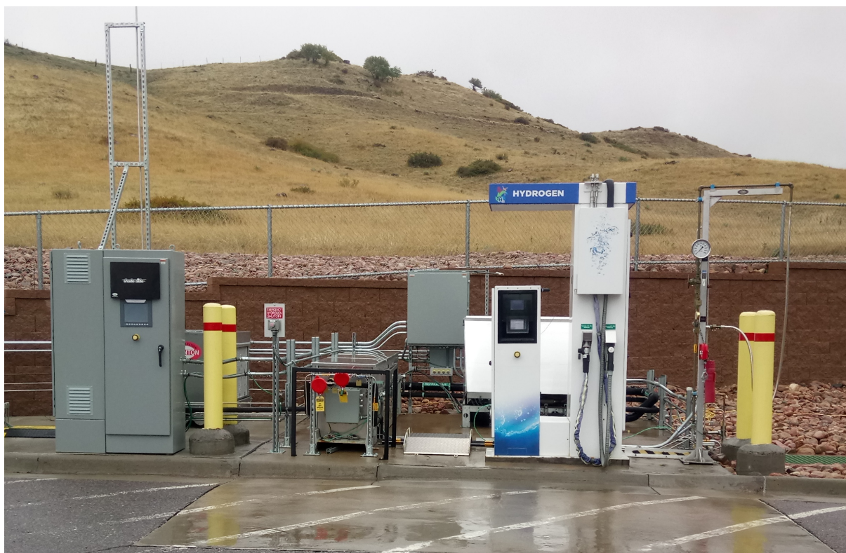
Figure 15. Hydrogen filling station at National Renewable Energy Laboratory, Colorado
