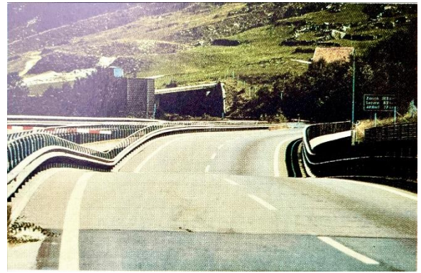
Picture 3: Superstructure lowered by 1.2 m and rotated counterclockwise
