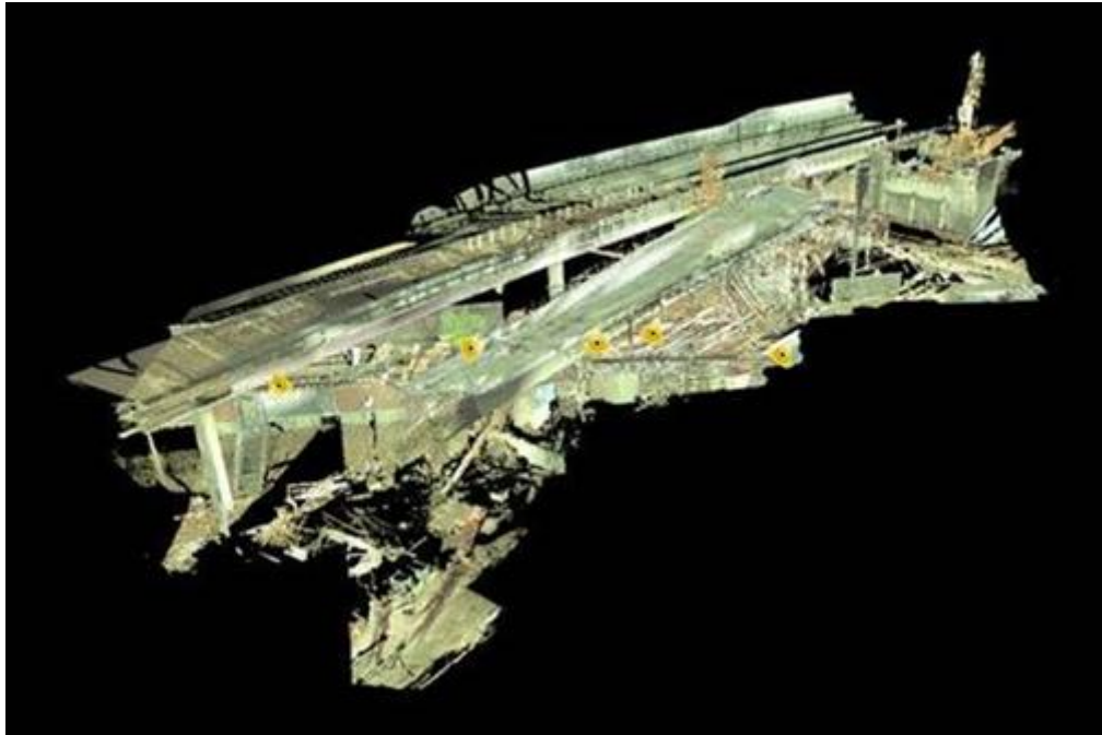
Figure 9: LIDAR point cloud documenting the position of the F3 Murbrücke Frohnleiten Bridge wreckage which collapsed in Austria on February 21, 2015.
