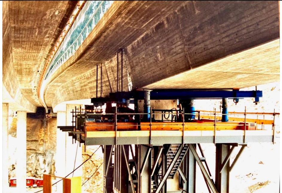
Picture 9: Lifting setup, detail. The blue beams and hanging rods are part of securing the broken beam.
