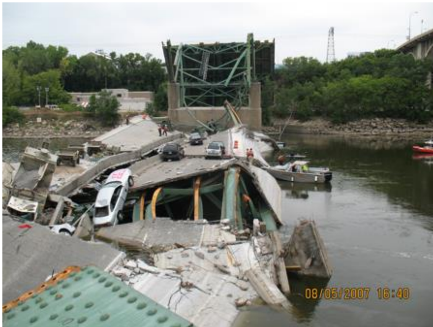
Figure 1: Wreckage of the I-35W Saint Anthony Falls Bridge which collapsed into the Mississippi River in Minneapolis, Minnesota, USA, on August 1, 2007.
