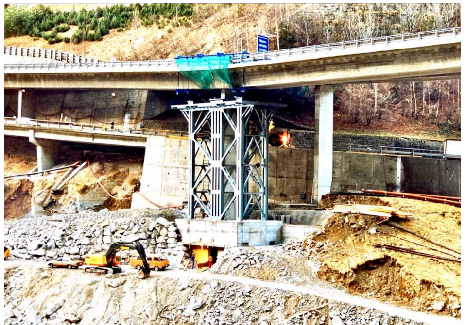
Picture 9: Reverse displacement device in place before lifting operation. Pilar J with new foundation.
