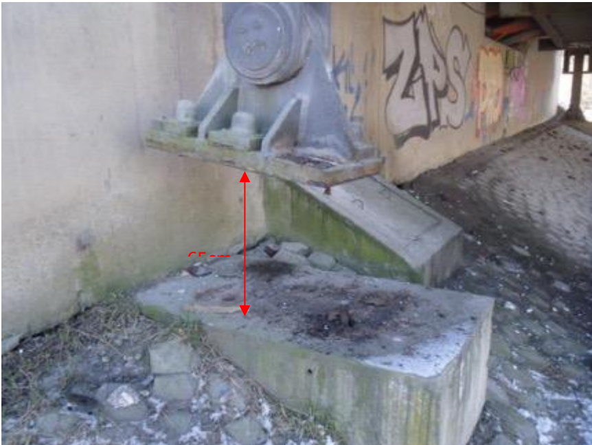
Picture of the support before failure
