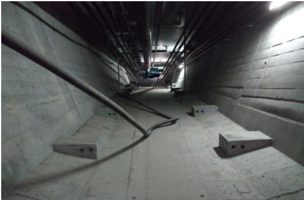
Figure 2: Photo of a failed post-tensioning tendon inside the Ré Island Bridge outside La Rochelle, France, on September 13, 2018.
