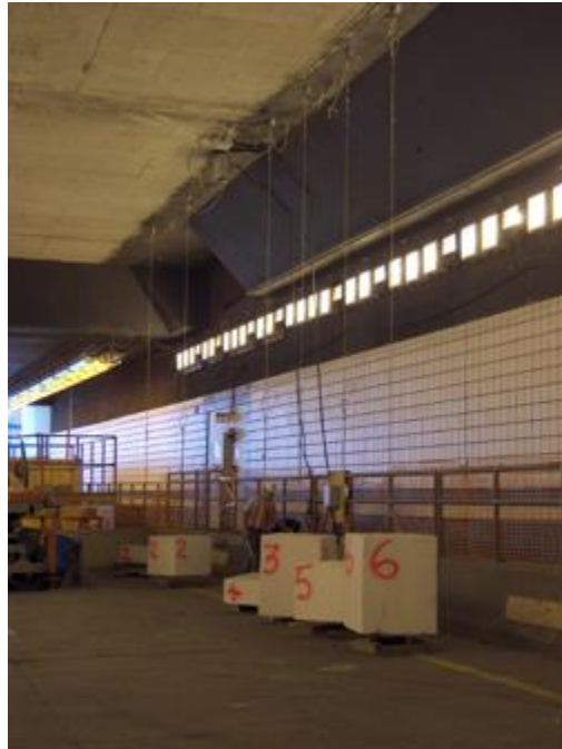
Figure 18: On-site sustained load testing of post-installed adhesive anchors.
