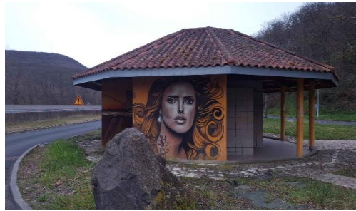
Covering graffiti with artistic paint in a rest area sanitary room-Photo 4 DIRMC
