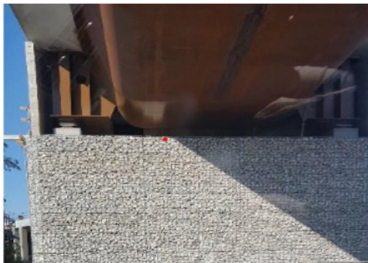
Gabion in front of concrete abutment of a mixed bridge
