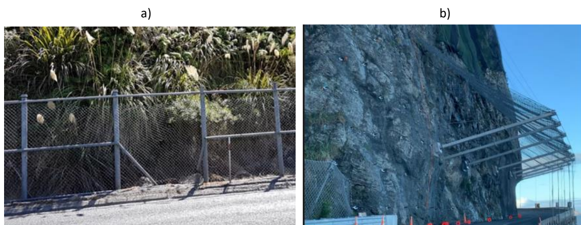
Figure 3.15 Examples of a rockfall protection in New Zealand; a) a road fence; b) the suspended mesh and cable nets in and around Kaikōura; ©NZTA.
