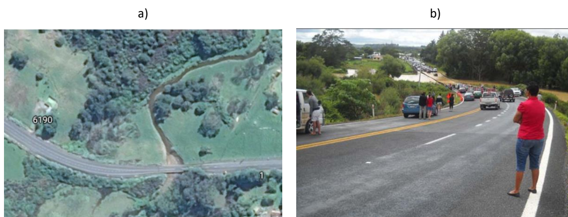
Figure 3.13 Flooding at Otiria Stream, Moerewa, New Zealand; a) aerial view of the site; b) a moderate flood event overtops a bridge; ©NZTA.
