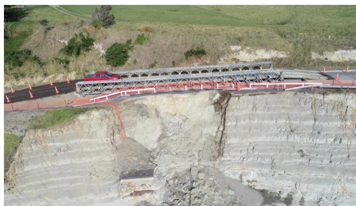
Figure 6.14 Application of a Bailey bridge at a landslide site on the Mahia East Coast Road, Wairoa District Council, 2019; ©NZTA.
