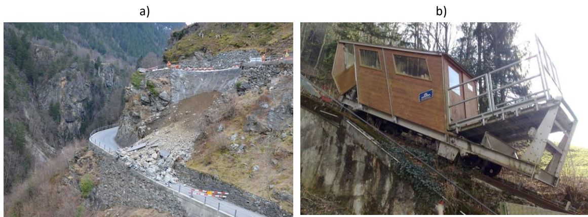
Figure 5.5 Mitigation of consequences of a road failure; a) Landslide at the Bristenstrasse, ©Canton of Uri; b) the old funicular railroad re-opened to transport passengers, ©Amsteg SBB power plant.
