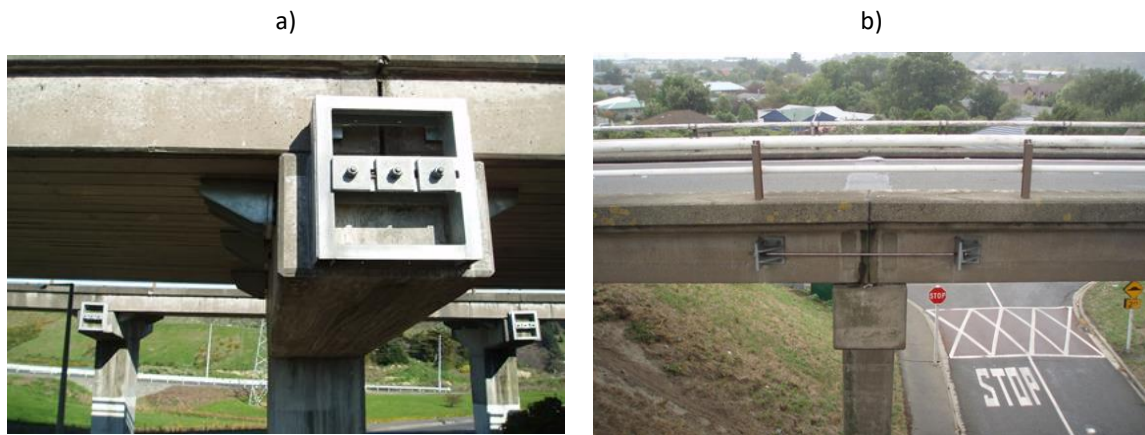
Figure 4.7. Examples of earthquake retrofit solutions on State Highway bridges in and around Christchurch, New Zealand. a) a shear key detail; b) a linkage bar detail; ©NZTA.
