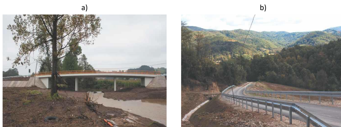
Figure 6.18. Reconstruction of assets after the flood in Serbia; a) reconstructed bridge on Jadar River in 2017; b) rehabilitation of “Vinjište” landslide in 2018, [69].
