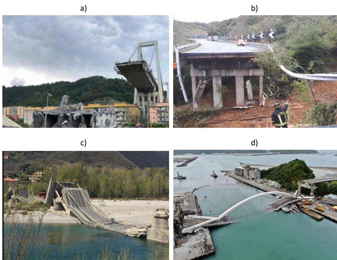
Figure 1.2 Recent bridge failures; a) Polcevera viaduct in Genoa, Italy (Aug.14 2018), @Vigili del fuoco.tv; b) Bridge on the A60 highway on Nov. 24 2021, Italy, @Vigili del fuoco.tv; c) Ponte di Caprigliola, Toscana, Italy (Apr.8 2020); d) Nanfang'ao Bridge, Yilan, Taiwan (Oct.1 2019), @CNA Photo (taiwannews.com)
