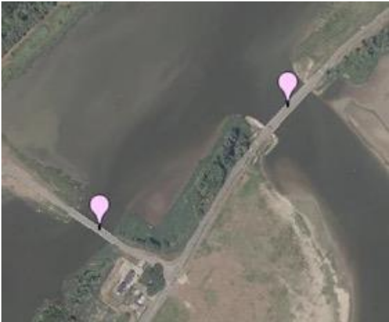
Bridges over breached dikes in the Biesbosch (Noordwaard project)
