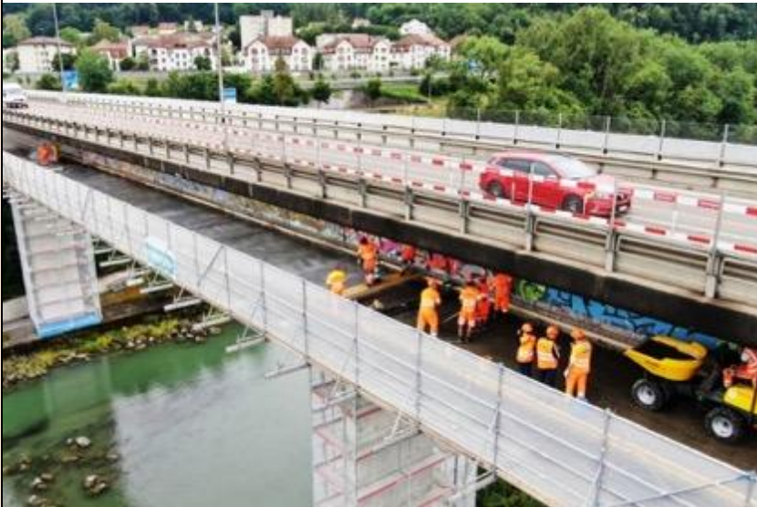
Application of the first layer on the lower deck
