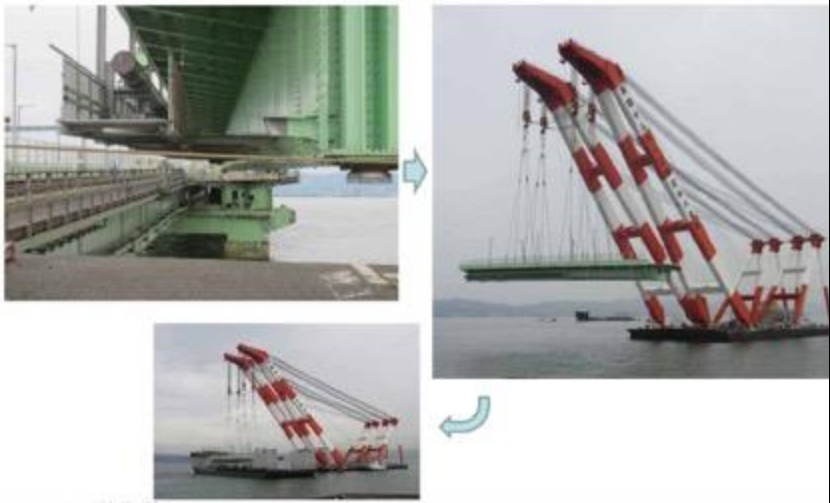
Removal of Girder by FC Vessel
