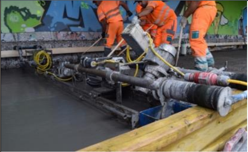
“Tremix” concrete vibrating beam in use on lower deck
