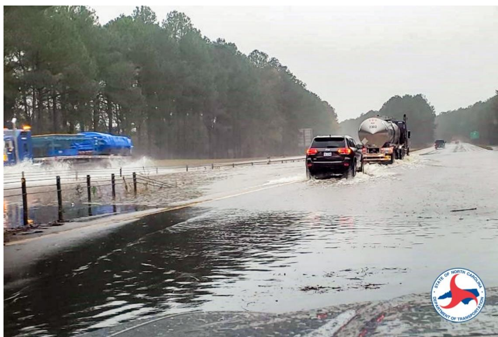
Figure 7.2.1-1: I-95 Flooding, 11-12-2020 (photo: Greg Dean, ACPA)
