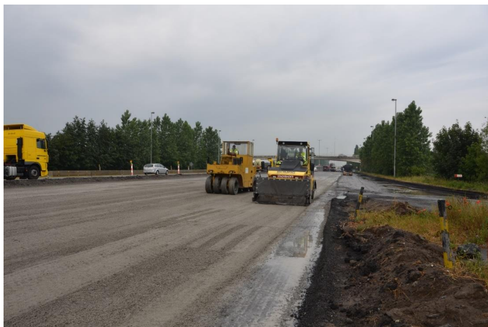
Figure 7.3.1-1: cement-bound base layer, A14, Belgium, 2011 (photo: Luc Rens)
