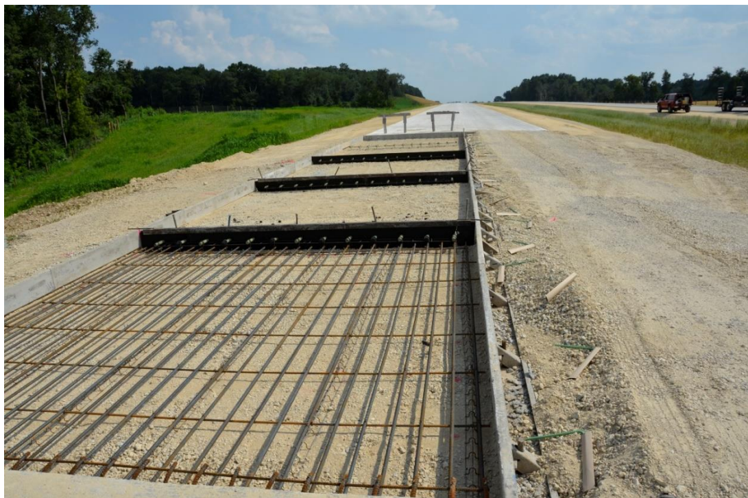
Figure 7.2.4-1: a series of expansion joints at the end of a jointed concrete pavement, Wisconsin, USA (photo: Luc Rens)
