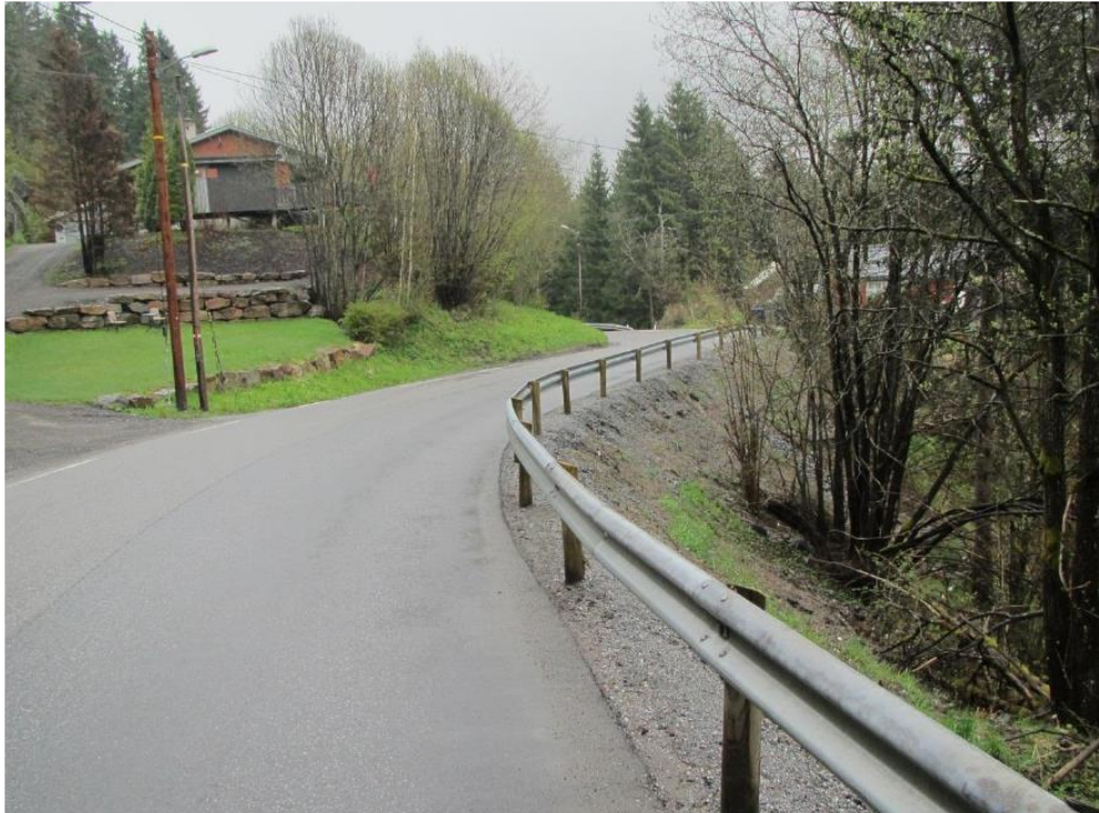
Figure 57: After strenghtening with foamglass and geogrid (Photo: Jan Vaslestad)
