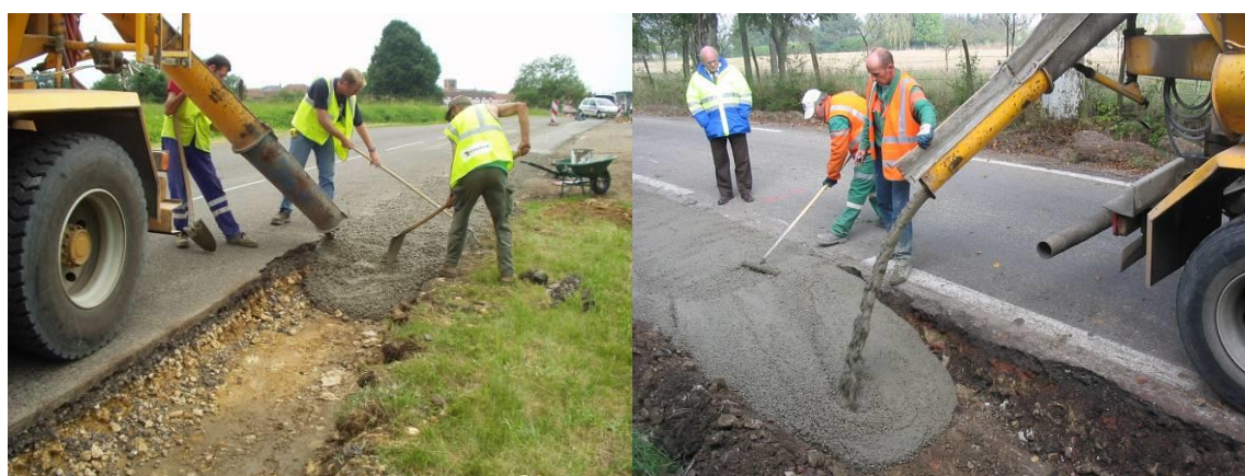
Figure 47: The material MACES is simply poured from truck mixes (left: RD 952 in 2003; right RD 19C in 2006)
