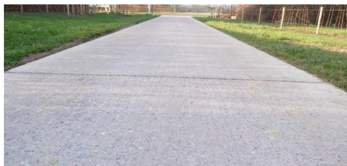
Figure 73 : Hasselt, BE – surface of a local road after micromilling (©Topoff, Belgium)
