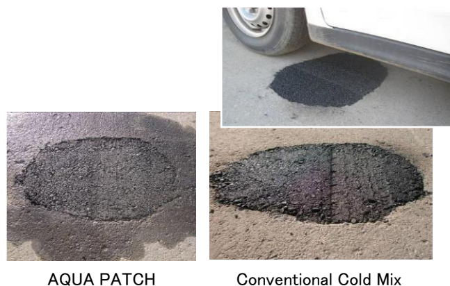
Figure 18: Durability immediately after repair work
