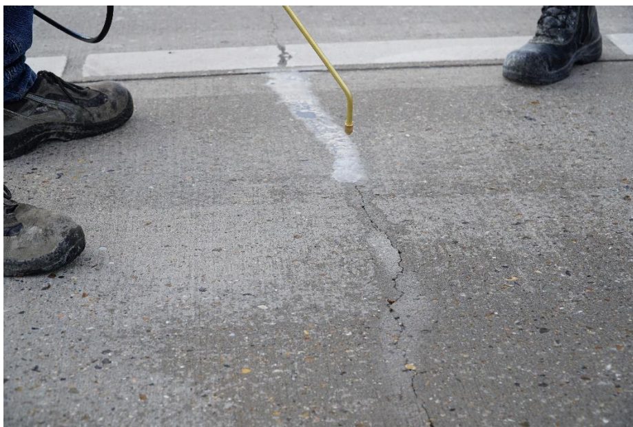
Figure 75 : Application of the repair liquid on a crack
