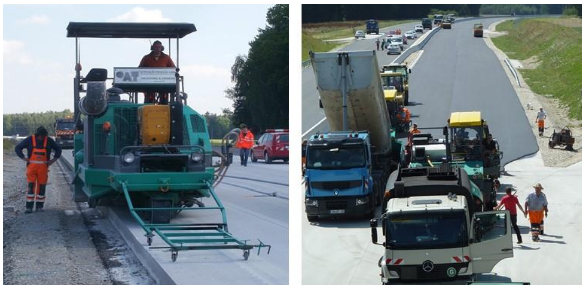
Figure 62: Production of the grinding texture of the asphalt surface course (DSH-V)
