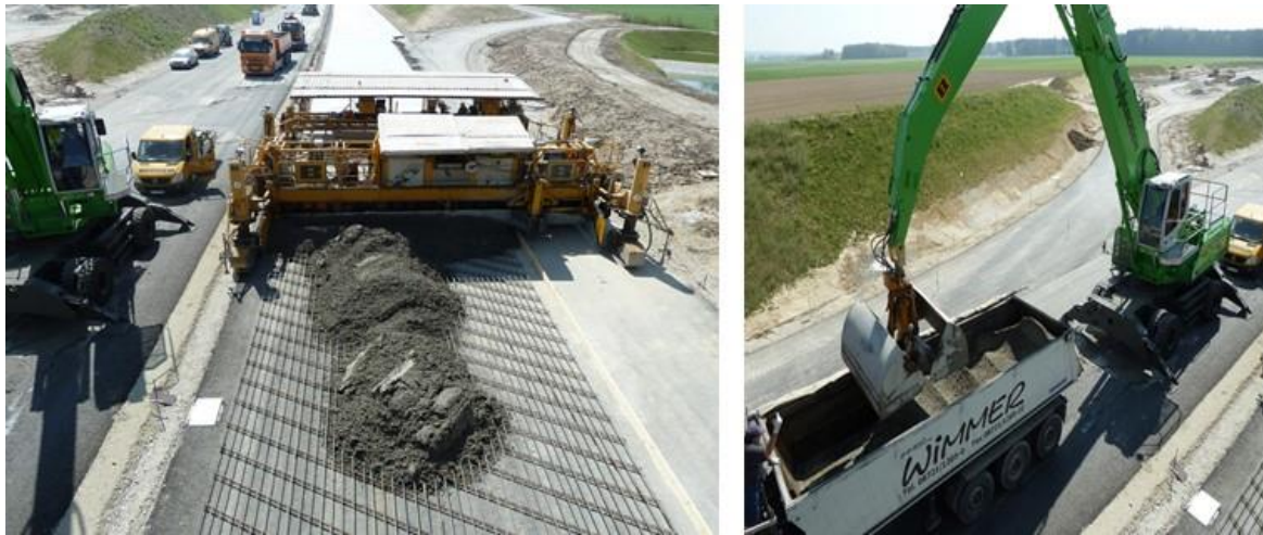
Figure 61: Concreting of the continuously reinforced concrete slab
