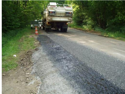
Figure 48: Surface dressing spread on the surface of the edge beam after setting
