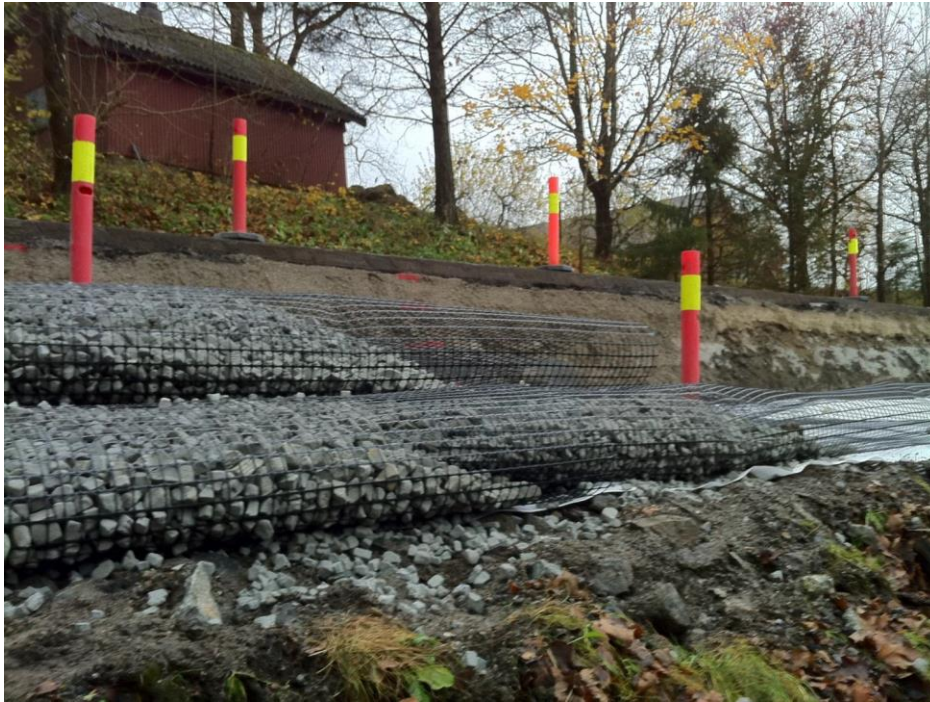
Figure 56: The geogrid is wrapped around the foamglass [4]
