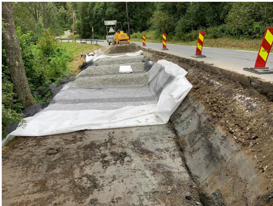
Figure 55: The next layers of foamglass is placed (Photo: Jan Vaslestad)
