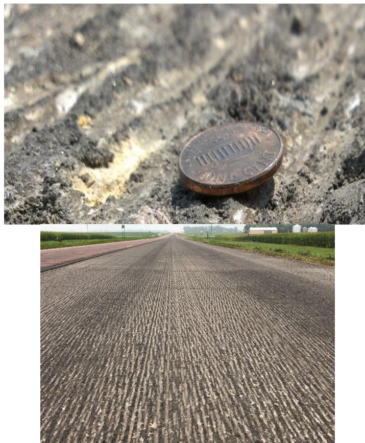
Figure 25: Micro Mill Photos: Finished micro mill texture and Micro Milled Pavement
