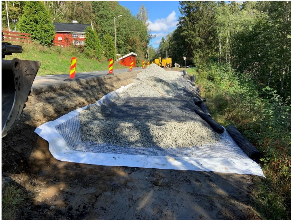
Figure 54: Nonwoven geotextile, geogrid and 40 cm foamglass is placed [4]
