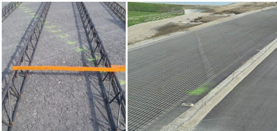
Figure 60: Placed transverse and longitudinal reinforcement
