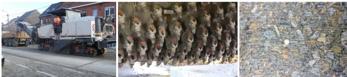
Figure 69 : Fine milling- from left to right: milling machine – rotating drum equipped with picking tools – result of surface after finemilling (©L. Rens, FEBELCEM)
