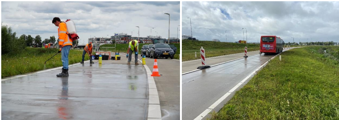
Figure 76: Surface application on a bus lane
