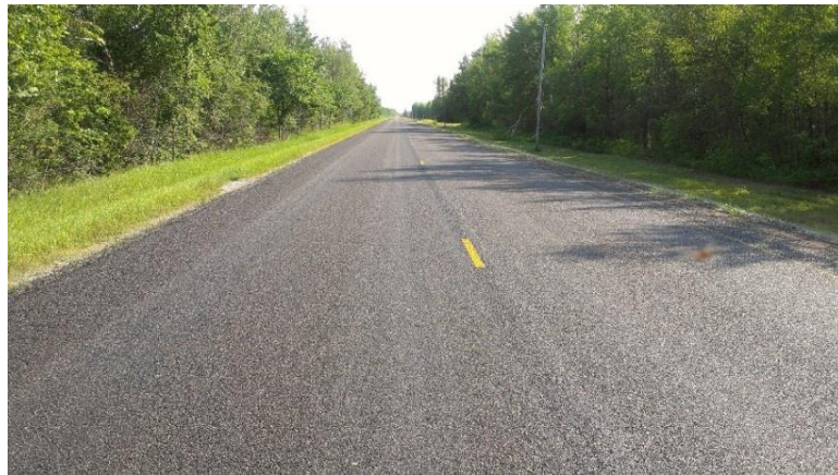
Figure 26: TH 89 after placement of chip seal (2013)
