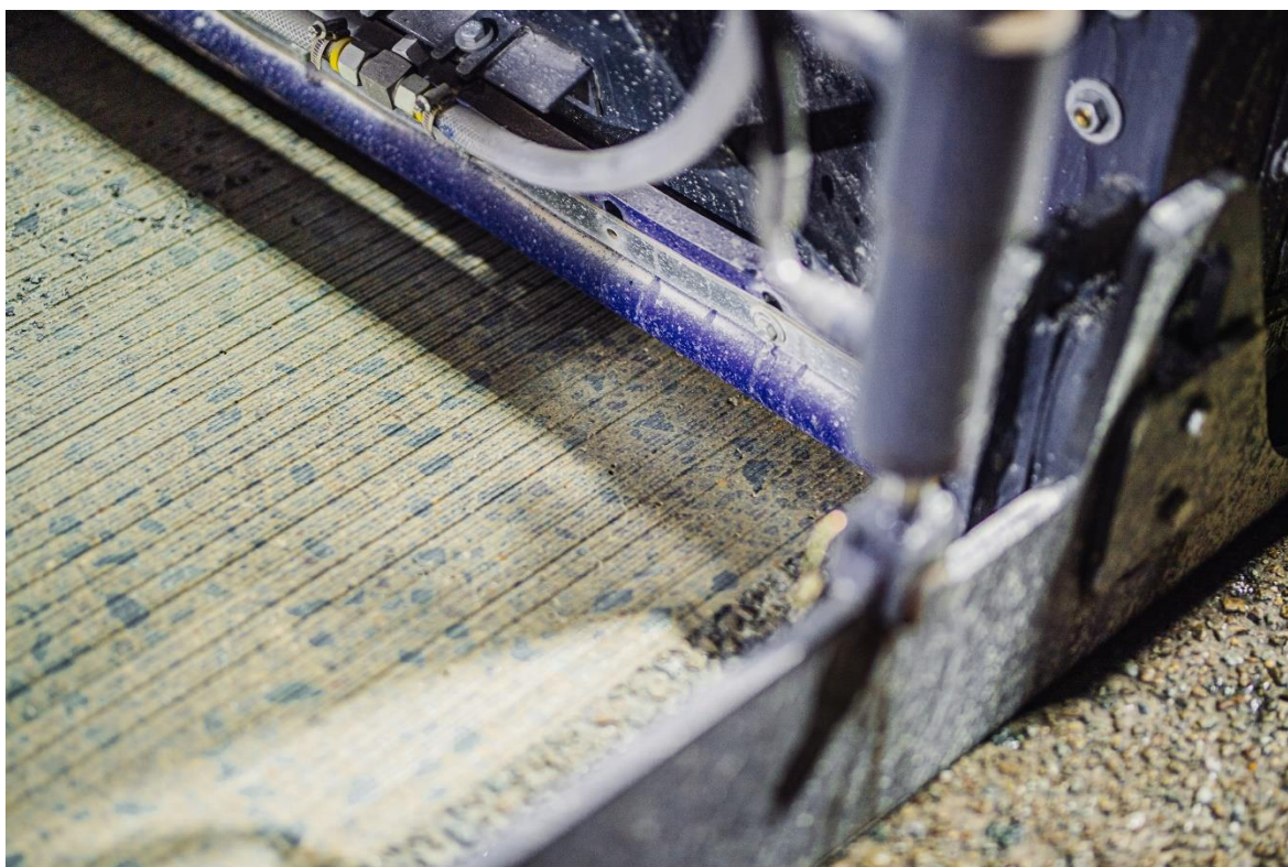
Figure 81: application of the NGCS profile on the R1 (picture by Kris Van de Sande, Agency for Roads and Traffic)
