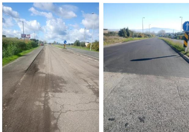
Figure 88: Typical punctual sanitation works before and after
