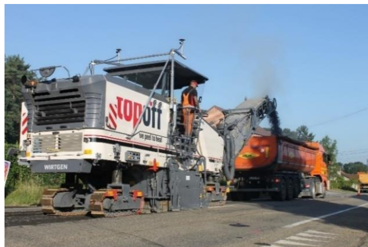
Figure 8: Milling machine with GPS antennas
