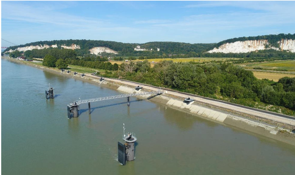
Copyright: Grand Port Maritime de Rouen The back-up emergency berth in Radicate (Rouen)
