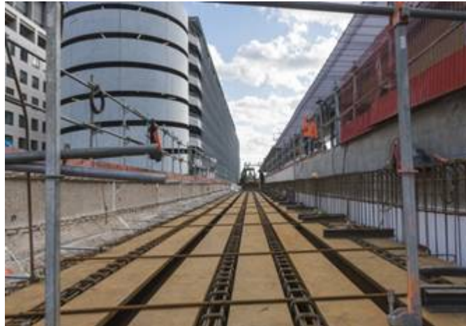
Action 2017-FR-TM-0013-W: the 12th platform track at Lyon Part-Dieu station (Source: SNCF Réseau)
