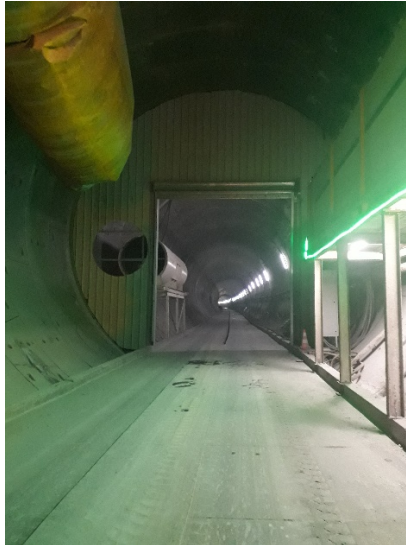
Action 2014-EU-TM-0401-M: entry of the first 9 km of the first tube of the tunnel (Source:INEA)
