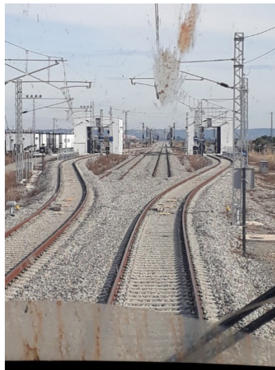
Action 2014-ES-TM-0438-W: Gauge changer along Valencia-Barcelona line (Source: INEA)
