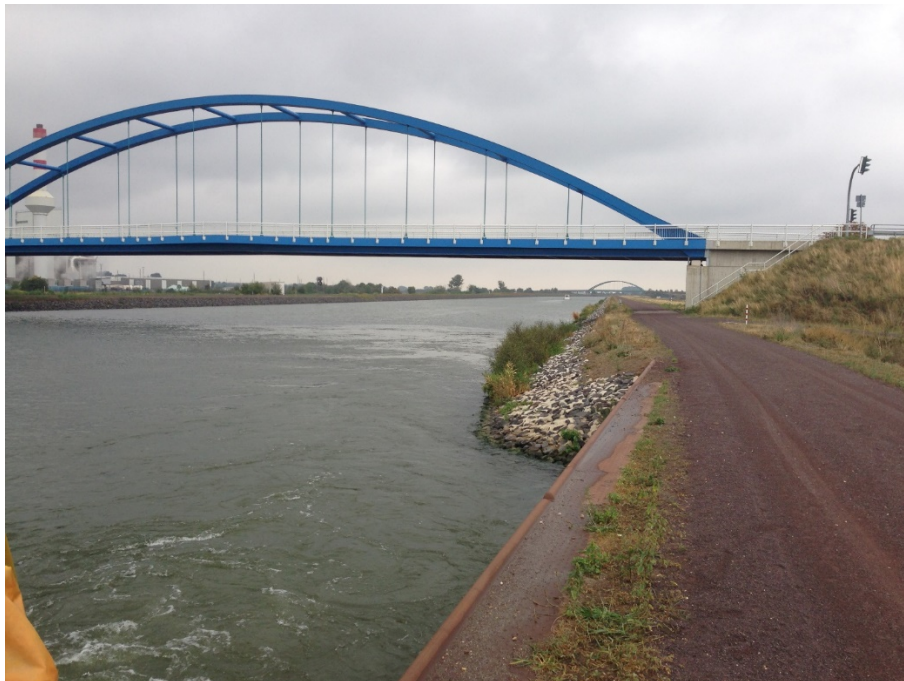
Extension of the Mittelland canal (MLK) from km 302.377 to km 303.800 is completed (Source: INEA)
