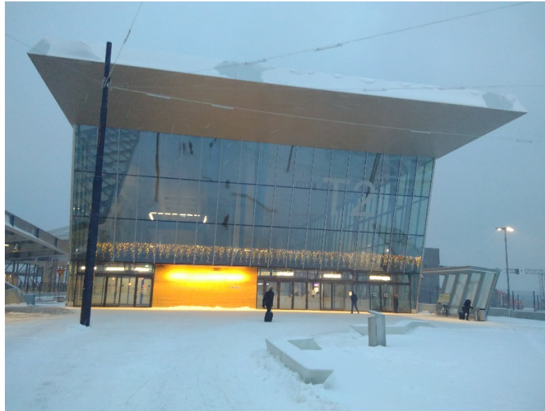
Developments in the T2 passenger terminal of Port of Helsinki were supported through CEF (Source: INEA)
