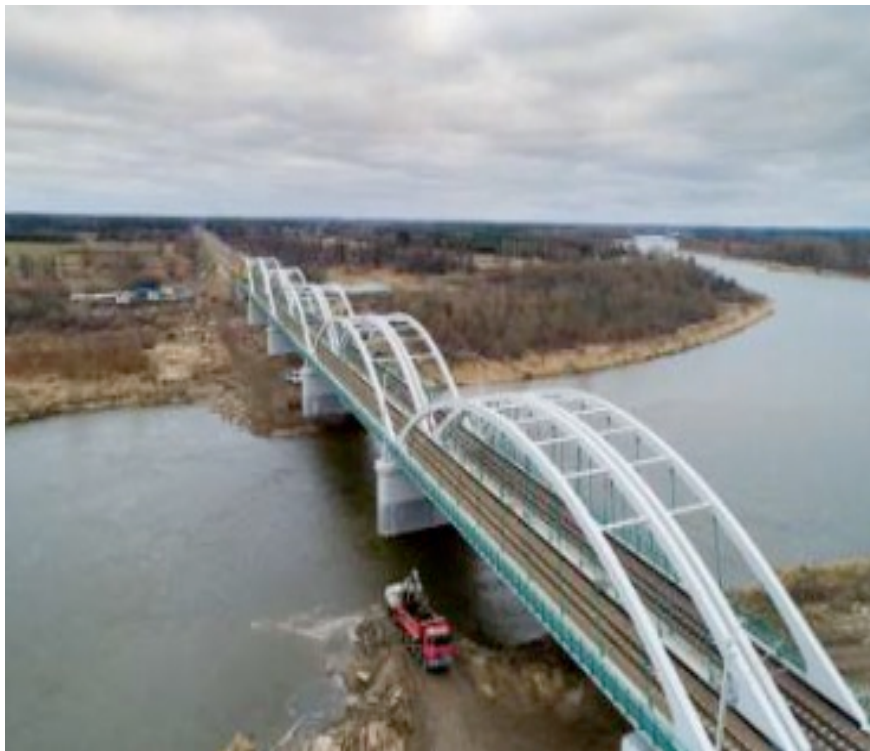
Bridge over river Bug in Poland, double track construction (Source: PKP-PLK SA)
