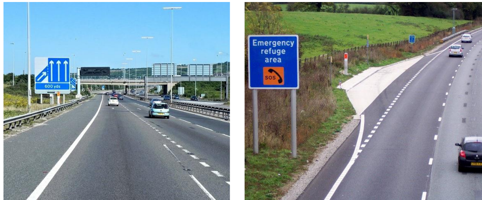
Figure 13 : Example of continuous hard shoulder (left) and Emergency Refuge Area (right)
