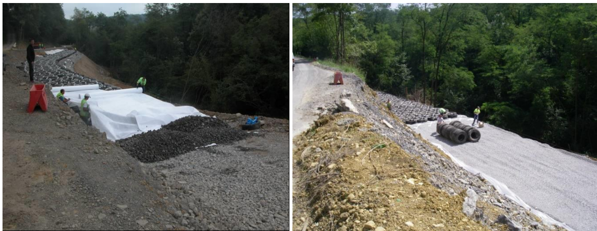
Figure 2 : Assembly line for Pneusol process – placement of tires and geosynthetic sheets and stockpile of gravel
