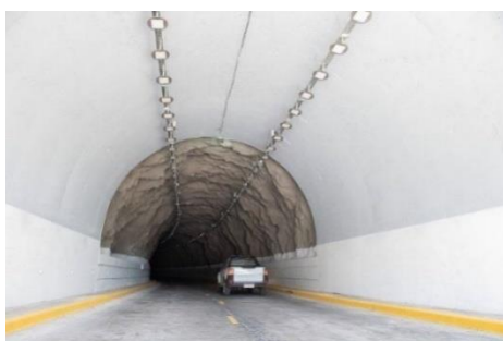
Photo 5 - overview the gallery of the tunnel after the works
