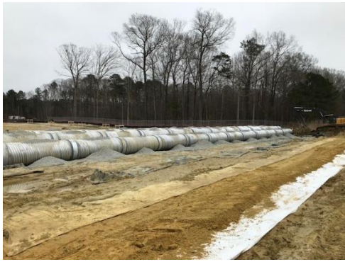
Figure 1 Installation of Temporary Culvert Pipes
