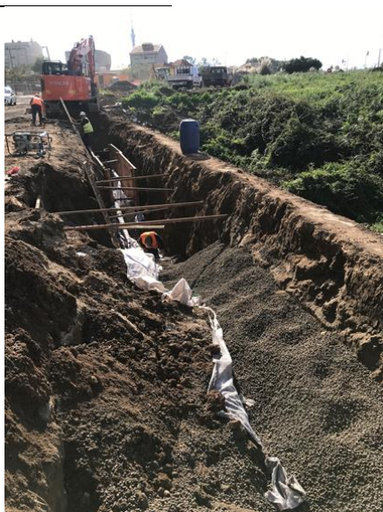
1.4 – Landfill during construction
