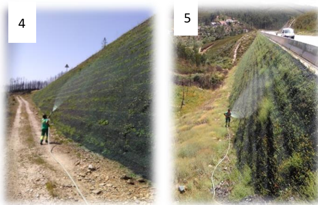
Figure 3 – Construction Phase 2017: Photos: 4) and 5) Hydroseeding works
