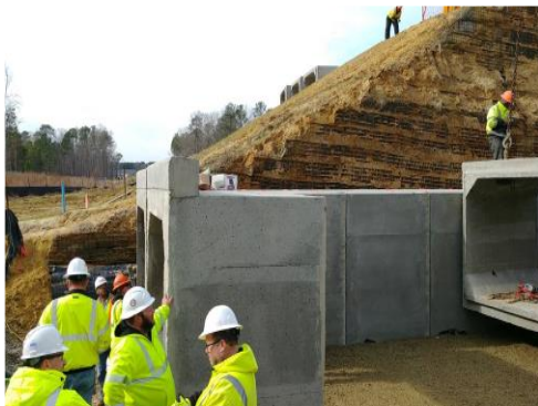
Figure 3 Placement of Precast Concrete Culvert Section Figure 4 Completed and Backfilled Culvert.
