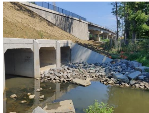
Figure 3 Placement of Precast Concrete Culvert Section Figure 4 Completed and Backfilled Culvert.
