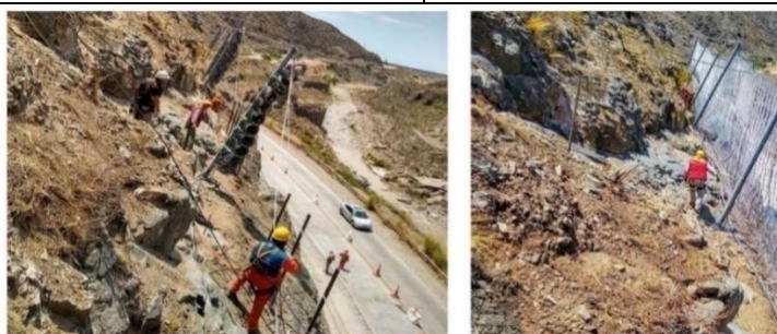
Photo 3 and 4 – works – debris flow protection barrier
