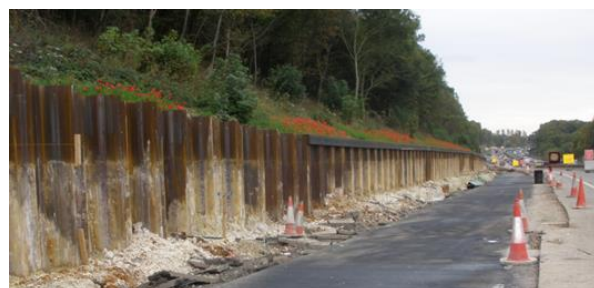
Figure 2: Completed King Sheet Pile Wall
