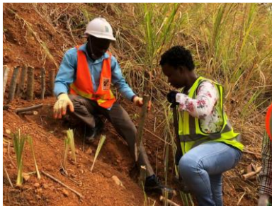
Figure 10: Live staking and fascines installation
