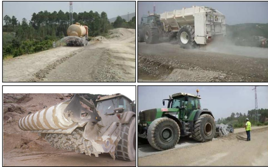
Construction Phase Photos (Clockwise from top left) – a) Placement of water, b) Addition of cement, c) Operation of mixer, d) Close up of mixer
