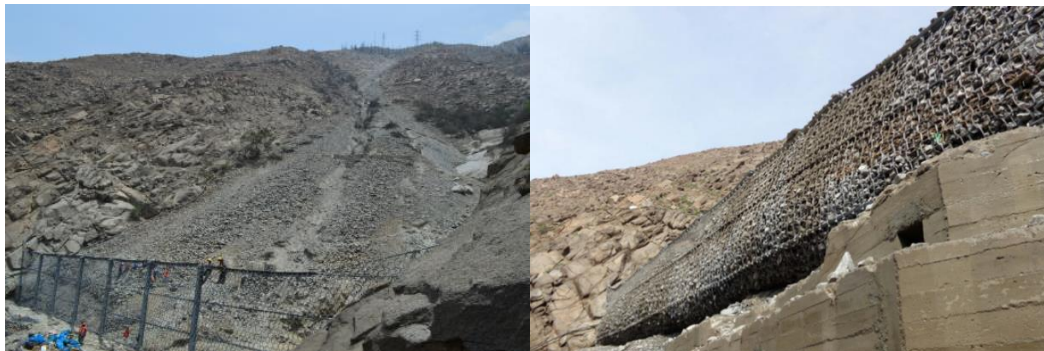
UX barrier instalation – Carosio Ravine (2016)
