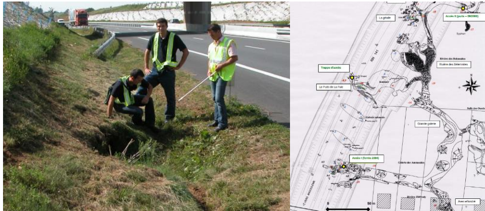
Figure 18 : inspection of LA FUIE cavity, RN.141, France (Courtesy Cerema)
