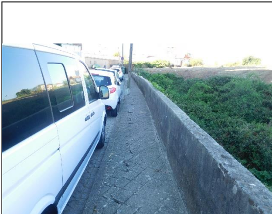
1.1 - Sidewalk and parking on top of the wall
