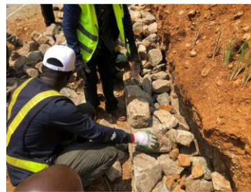
Figure 11: Construction of dry-stone toe wall
