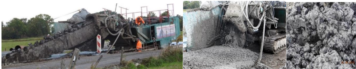
Pictures: The FMI (cut-mixing-injection) machine - Sidla & Schönberger Germany
