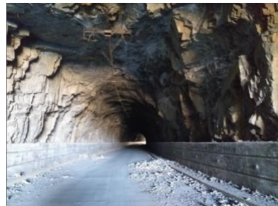
Photo 2 overview the gallery of the tunnel before the works
