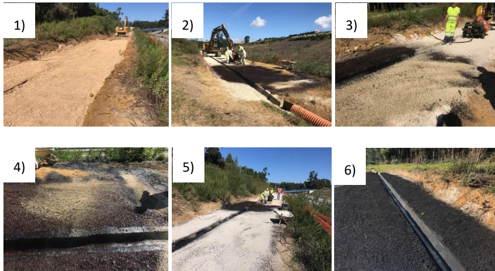
Figure 2 – Construction Phase: Photos: 1) Removal of all vegetation and removal of the landslide materials from the bottom of the excavation slope; 2) The installation of rockfill, 3) Stripping the entire length and width of the bank, with a thickness of 10 cm and 4 and 5) Waterproofing the excavation slope stool by applying a 10 cm thick granular rock aggregate + 1.5 cm thick double bituminous coating + 6 / 10 mm gravel 6) Final view after the intervention.
