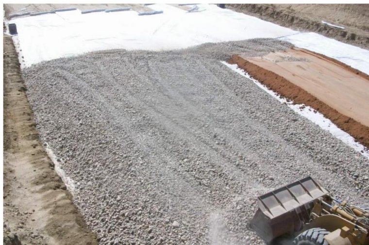
Figure 3. Granular drainage layer, geotextile and backfill layer
