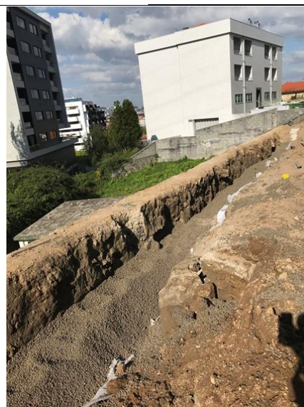
1.5 – Landfill during construction
