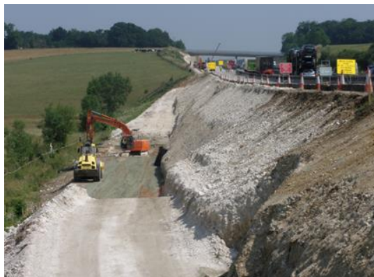
Figure 1: Embankment construction using glass sand
