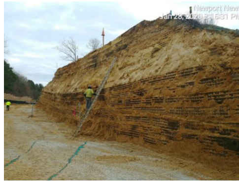
Figure 2 GSE Walls Being Used as Excavation Support.
