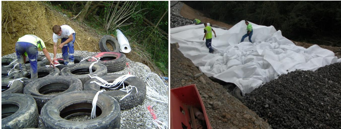
Figure 3 : tire bonding operation and then fitting the geotextile into the tire hubs
