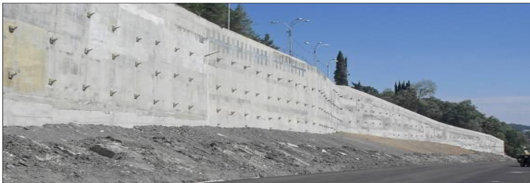
Figure 1. Pile anchor landslide protection structure at the interchange in the area of the city of Sochi
