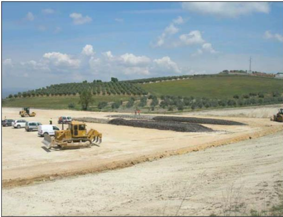
Fig. 1. Construction of experimental embankments made of shredded end-of-life tires (SEOLTs)
