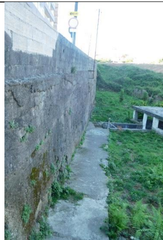
1.2 - Front view of the wall
