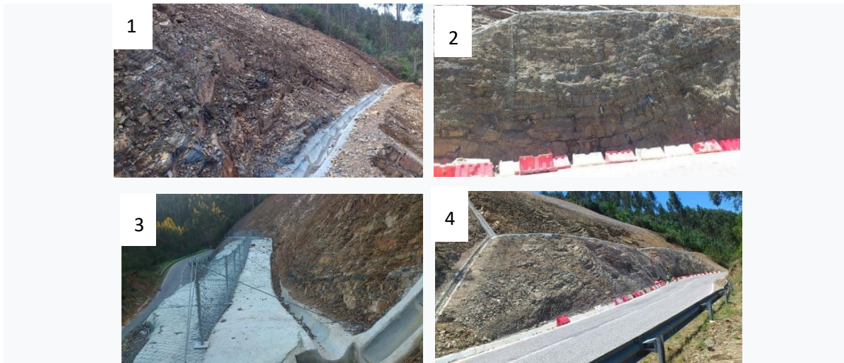
Figure 3 – Construction phase photos: 1) Earthmoving - Removal of unstable material and profiling of the cutting slope, 2) Application of metal mesh, 3) intermediate shoulder, 4) Final view.
