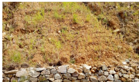
Figure 13: Grass and stone toe wall after three months
