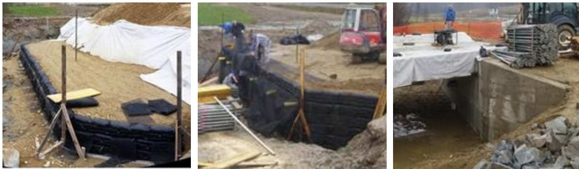
Photos 1,2 and 3 – construction phase
