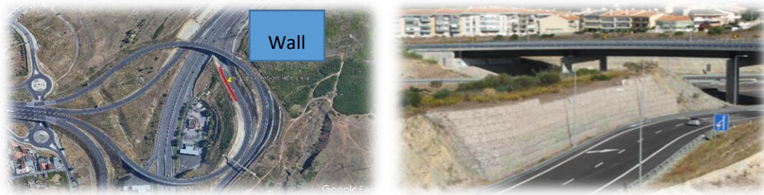
Figura 1: localization and longitudinal view of the gabion wall
